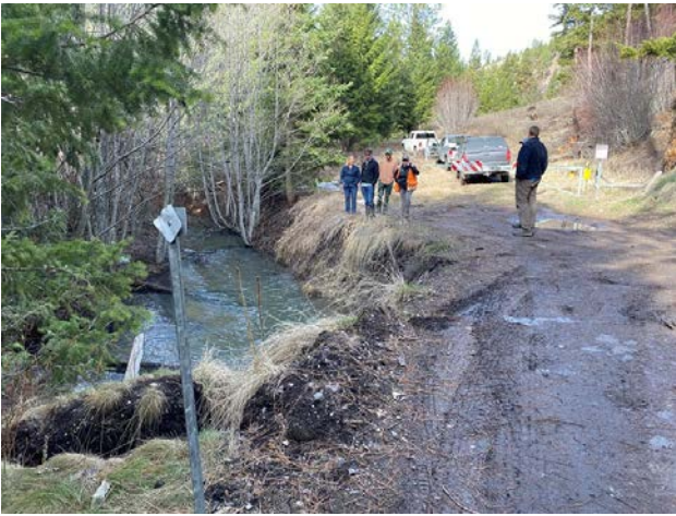
Figure 1. O'Brien Creek is eroding the stream-side roadbed at several locations. This picture shows an actively eroding section of roadbed the at the beginning of the restoration reach. The road will be re-located away from the stream, and vegetated wood matrix and large wood structures will be installed creating an inset floodplain.
