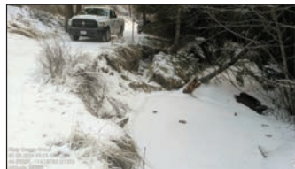
EXISTING CONDITIONS, UPPER O'BRIEN CREEK. LEFT: ROAD PRISM/FILLSLOPE EROSION AND BLOCK FAILURE. RIGHT: ENTRENCHED, SIMPLIFIED CHANNEL LACKING LARGE WOOD.
