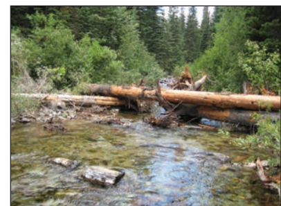
EXAMPLE CHANNEL-SPANNING LOG ARRAY
