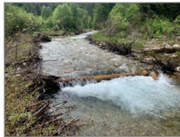
TYPICAL CONSTRUCTED STREAMBED THROUGH A RIFFLE FEATURE
