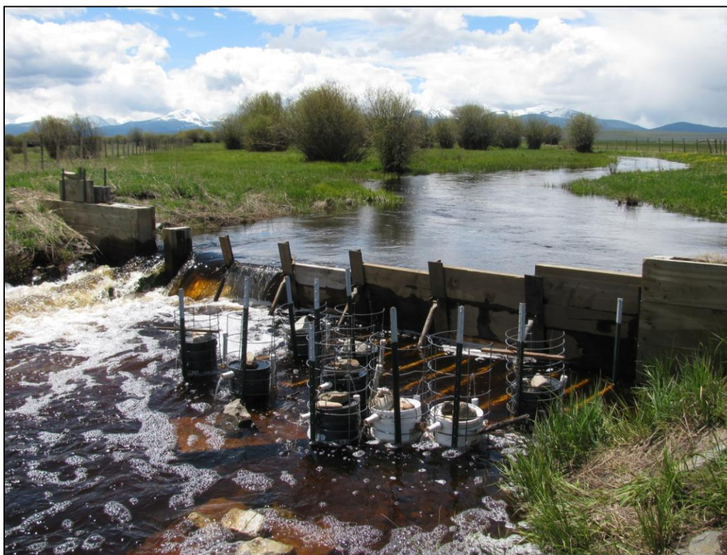
Figure 7. Remote site incubators were positioned downstream of existing pin and plank diversion structure to alleviate high flow conditions and provide backwater areas for fry.
