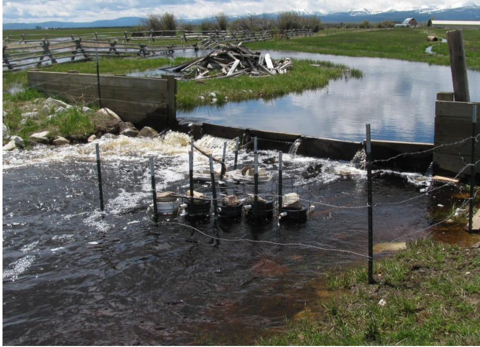
Figure 9. Remote site incubators were positioned downstream of existing pin and plank diversion structure to alleviate high flow conditions and provide backwater areas for emerging fry.
