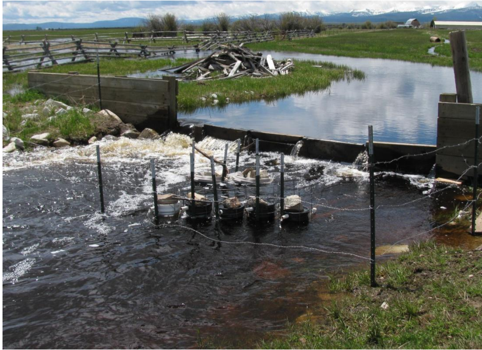
Figure 6. Remote site incubators were positioned downstream of existing pin and plank diversion structure to alleviate high flow conditions and provide backwater areas for emerging fry.
