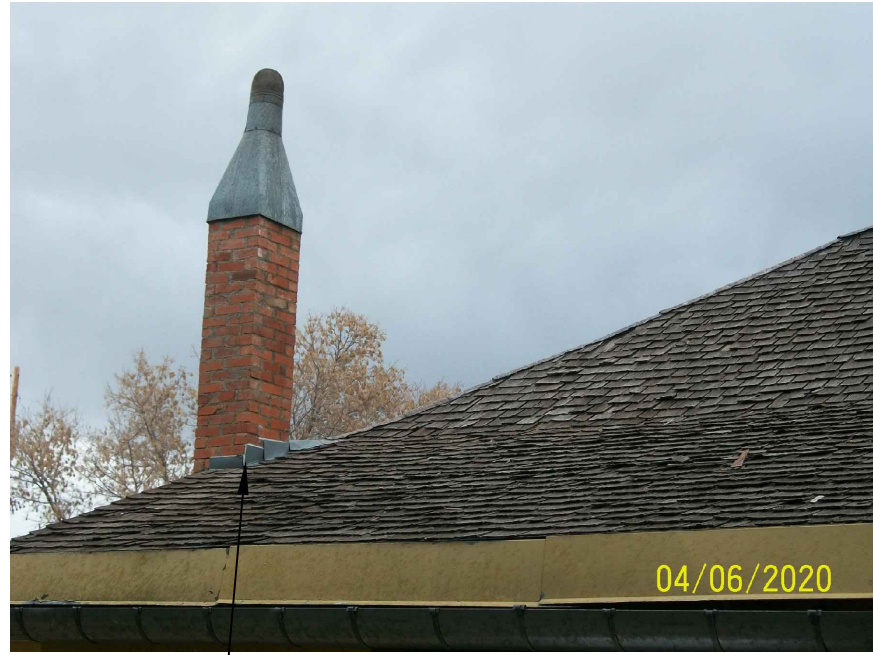
INSTALL GALV. BASE FLASHING UNDER EX. STEP FLASHING
