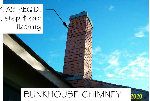
REPAIR DAMAGED BRICK & REPOINT AS REQ'D. install base flashing
