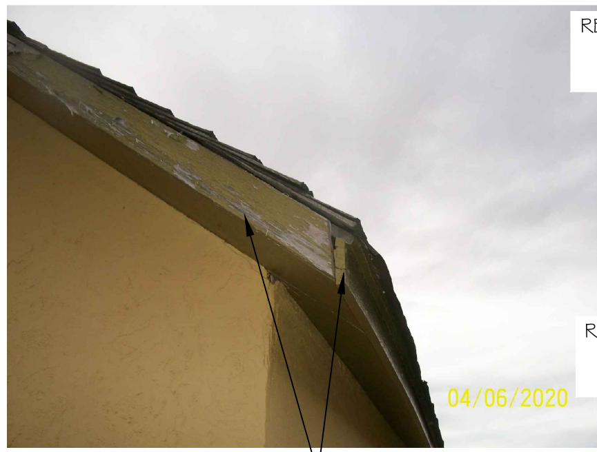
INSTALL NEW 1x FASCIA & GABLE TRIM BUNKHOUSE NORTH ELEV.
