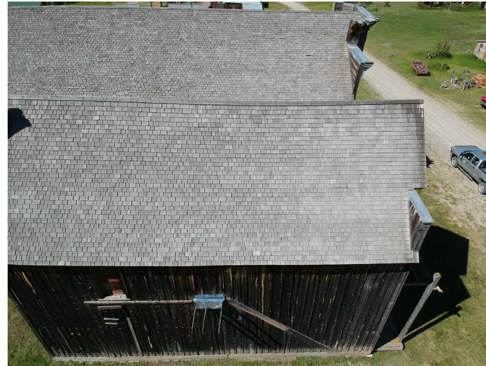
VIEW OF NORTHEAST ROOF SLOPE, FRONT OF BUILDING
