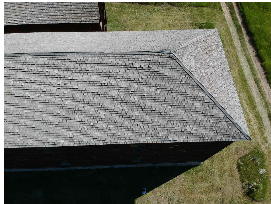
VIEW OF SOUTHWEST ROOF SLOPE, REAR OF BUILDING
