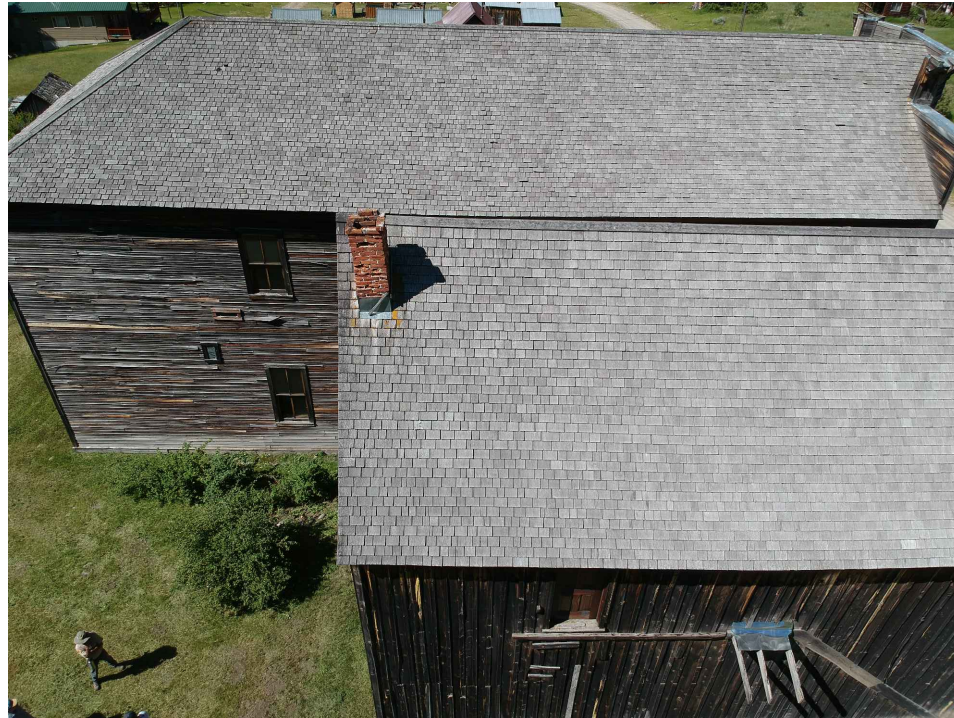
VIEW OF NORTHEAST ROOF SLOPE, REAR OF BUILDING
