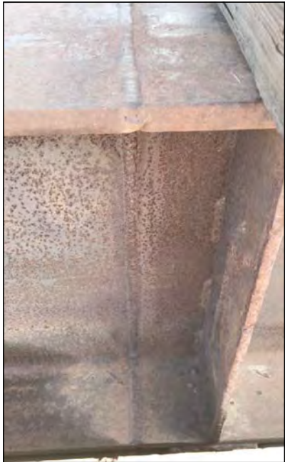
PHOTO OF EXISTING GIRDER SPLICE WELD
