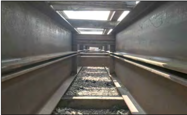
PHOTO OF EXISTING INTERMEDIATE STIFFENERS AND DIAPHRAGMS
