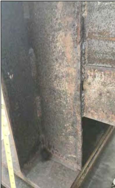
PHOTO OF EXISTING END STIFFENERS
