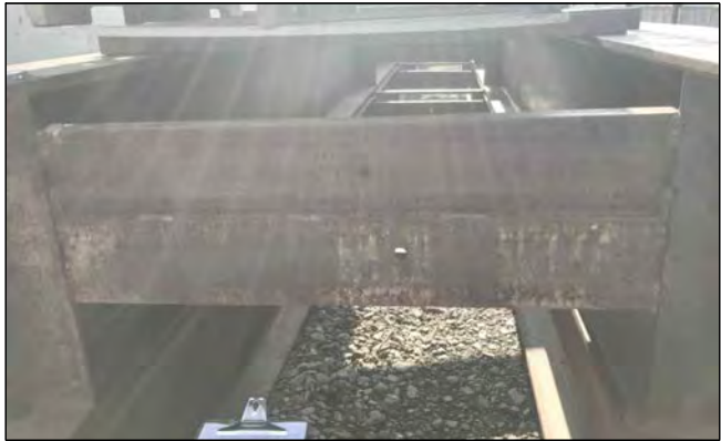
PHOTO OF EXISTING END DIAPHRAGMS
