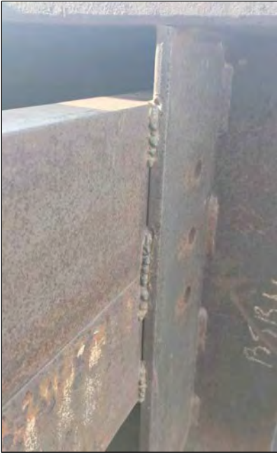
PHOTO OF EXISTING DIAPHRAGM WELDS
