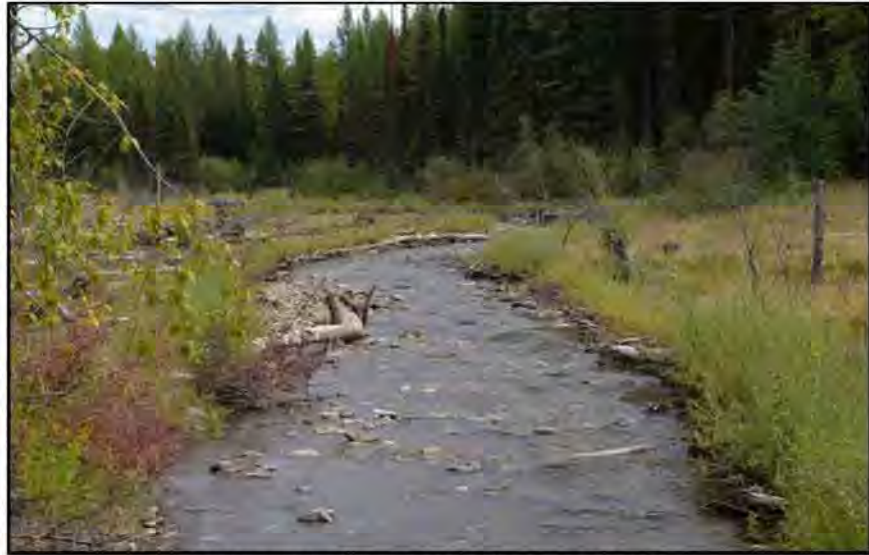
TYPICAL CONSTRUCTED STREAMBED THROUGH A RIFFLE FEATURE
