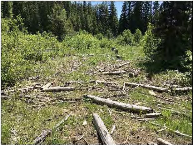
EXAMPLE OF CONSTRUCTED FLOODPLAIN ROUGHNESS
