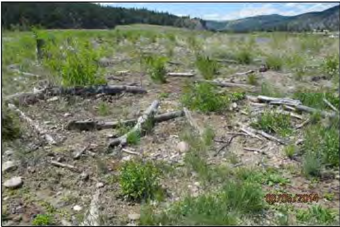
EXAMPLE OF CONSTRUCTED FLOODPLAIN ROUGHNESS
