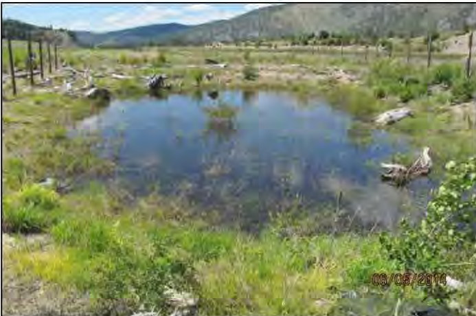
EXAMPLE OF CONSTRUCTED FLOODPLAIN SWALE
