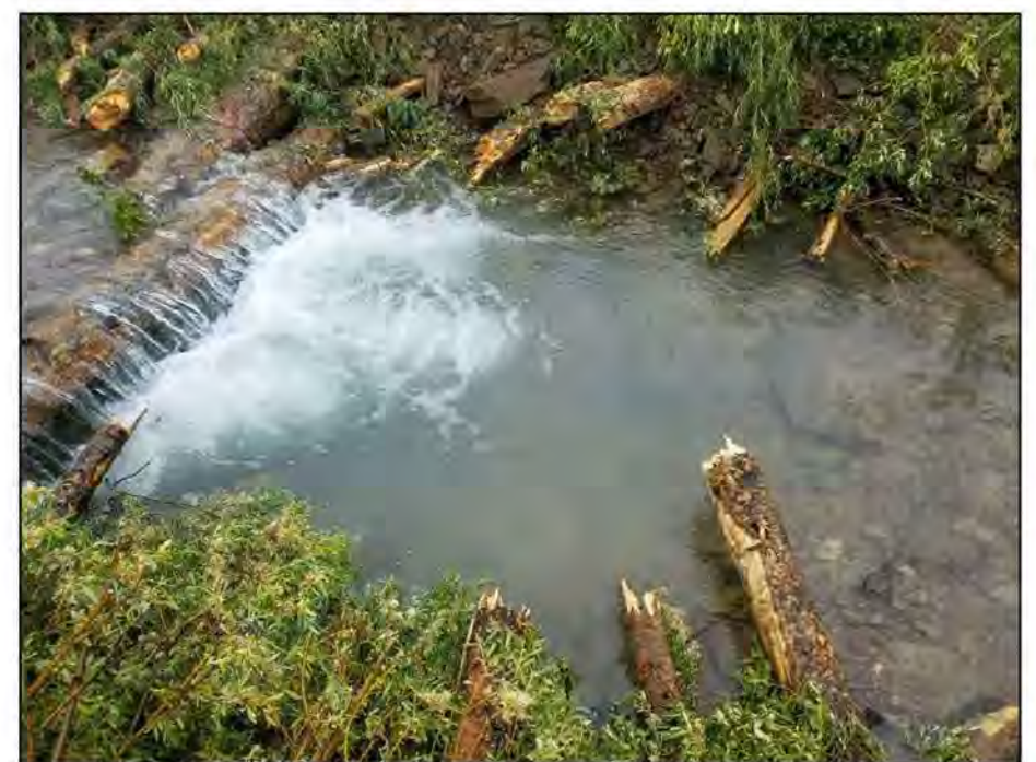
EXAMPLE OF A CONSTRUCTED LOG STEP POOL
