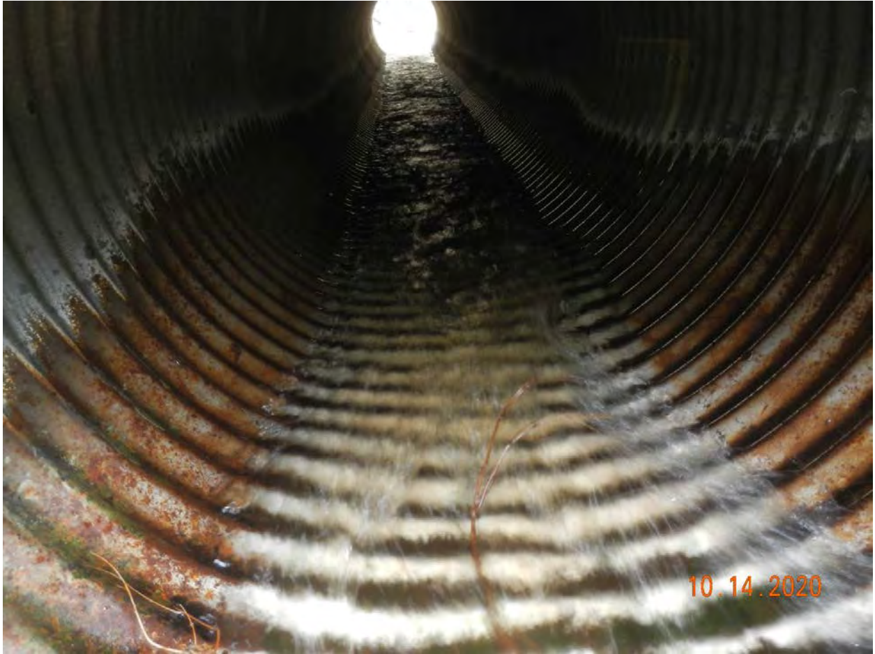
Looking downstream through the barrel of the Road 5771 culvert
