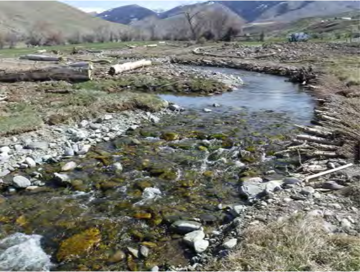
EXAMPLES OF CONSTRUCTED RIFFLE TREATMENTS
