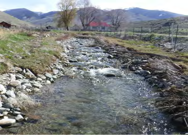
EXAMPLES OF CONSTRUCTED RIFFLE TREATMENTS
