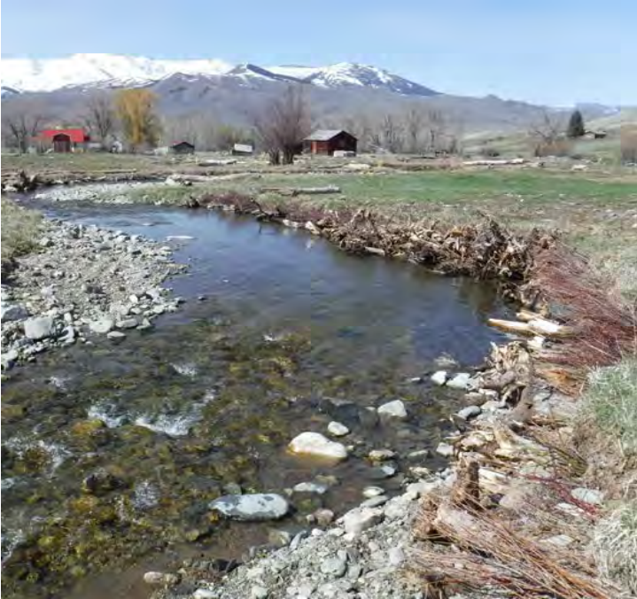
EXAMPLES OF LARGE WOODY DEBRIS STRUCTURE TREATMENTS
