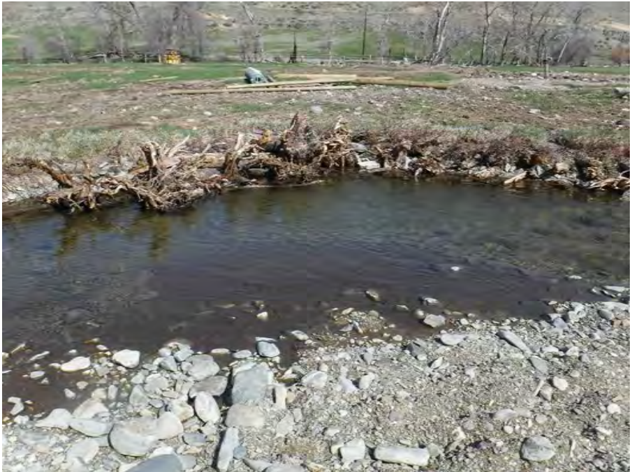
EXAMPLES OF LARGE WOODY DEBRIS STRUCTURE TREATMENTS
