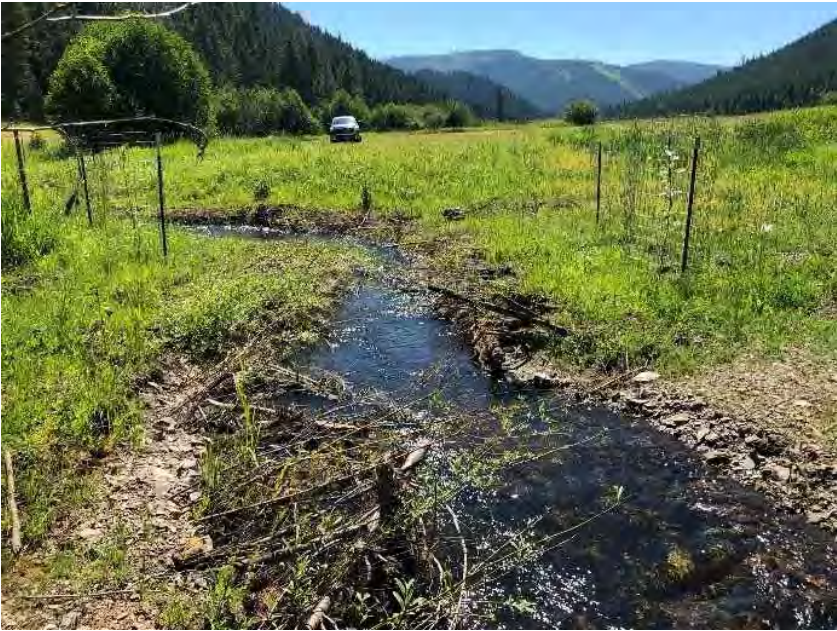
EXAMPLES OF WOODY DEBRIS MATRIX STREAMBANK TREATMENTS
