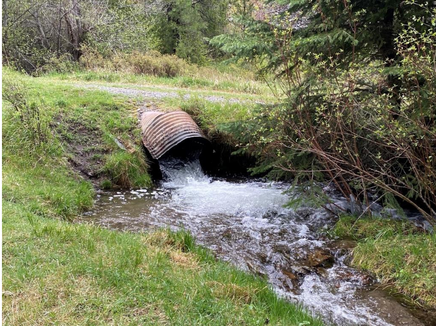
Figure 1: Little Park Creek perched culvert on TNC lands to be replaced with beneficial barrier.
