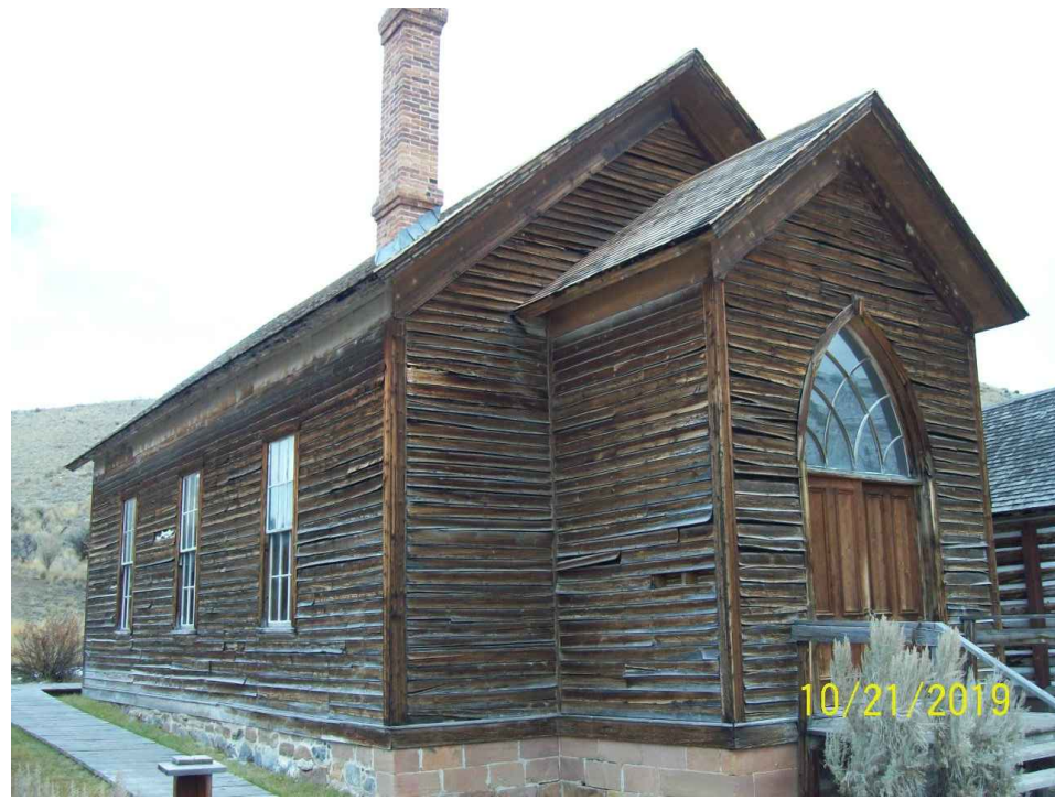
FRONT VIEW - LOOKING NORTHEAST
