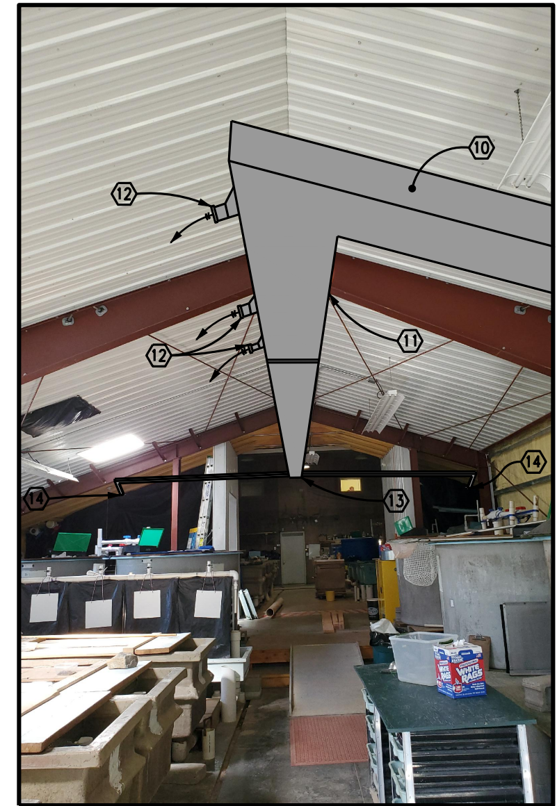
3 DUCT ROUTING ME-6 ADDITION NO SCALE
