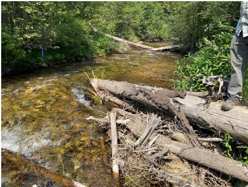
An example of the proposed treatment - a \frac{1}{2} spanning large wood jam installed along the Cedar Creek Road.
