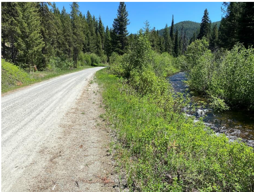
The East Fork Lolo road is chronically delivering sediment to the stream and limiting wood recruitment into the stream.
