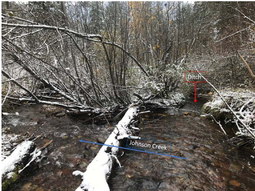
Photo 1: Standing in Johnson Creek looking downstream towards the Hammond Ditch inlet. Note the lack of check structure and headgate.
