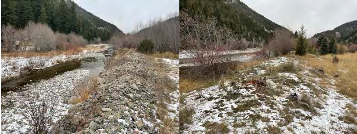
Figure 1: Photos of earthen berms that have cut off Mill Creek from its historic floodplain. The proposed project would breach these structures.
