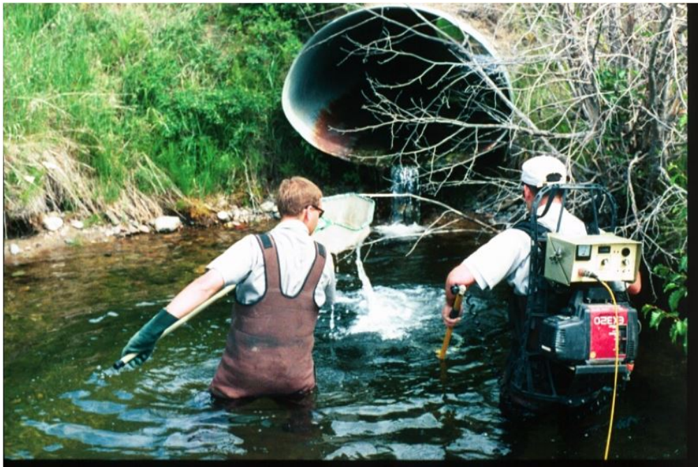
Figure 2. Perched Culvert on lower Murphy Spring Creek before replacement.
