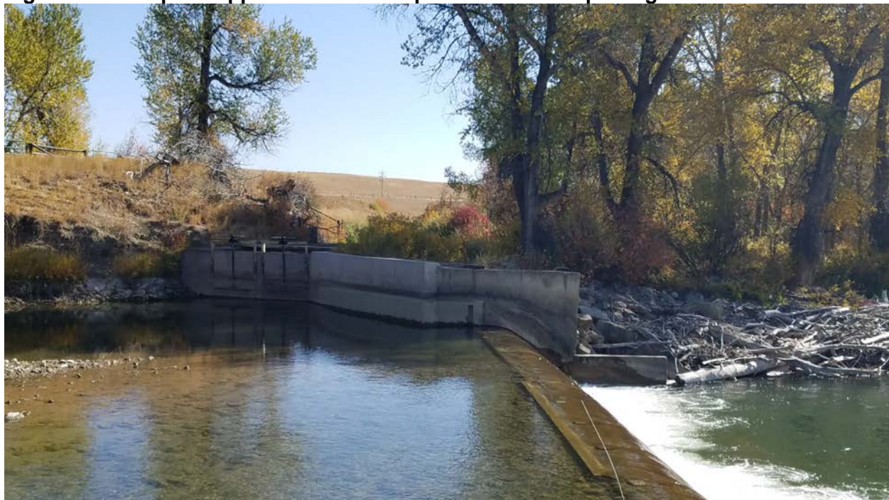
Figure 4. Wing wall on opposite side of diversion showing elevation of planned retrofit.
