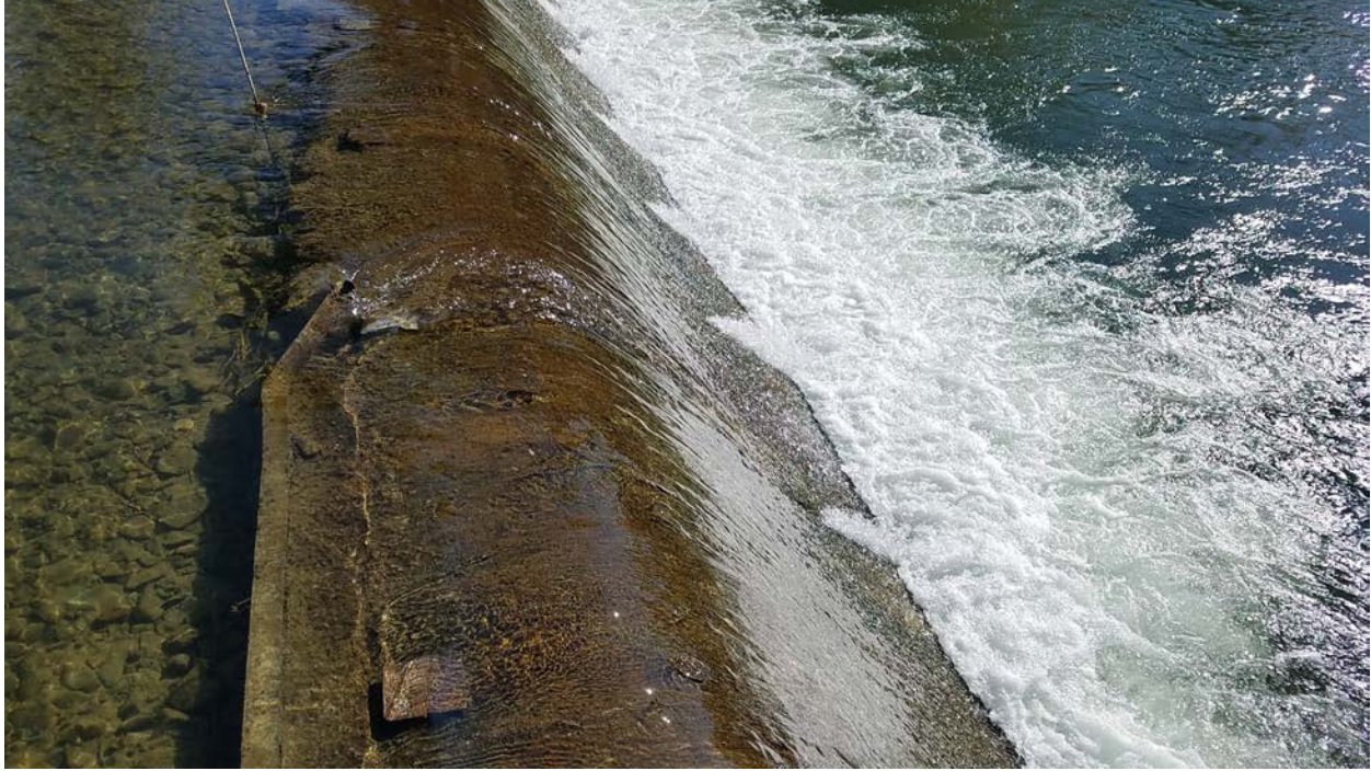
Figure 5. Spalling concrete and twisted angle iron on top of diversion.
