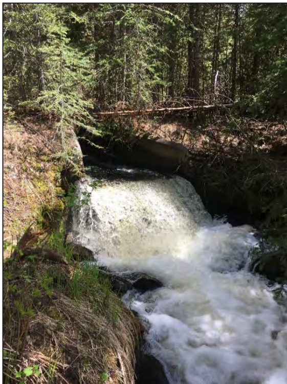
Figure 1. Perched culvert
