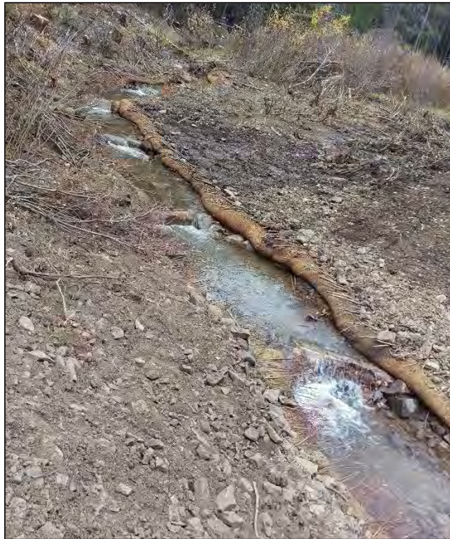
Figure 4 – Complete step-pools in lower French Gulch
