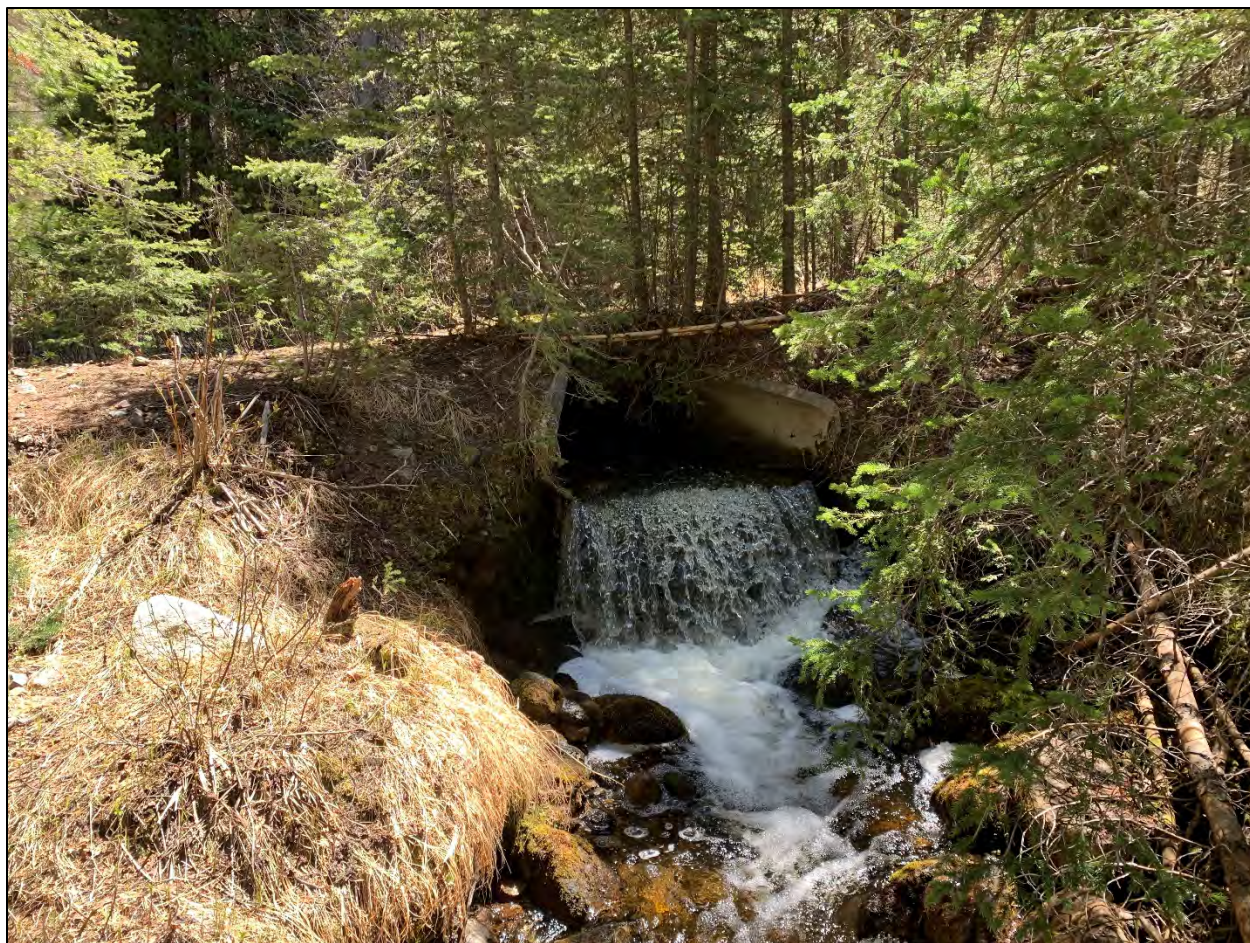
Perched culvert upstream of cascade. May 28, 2021.
