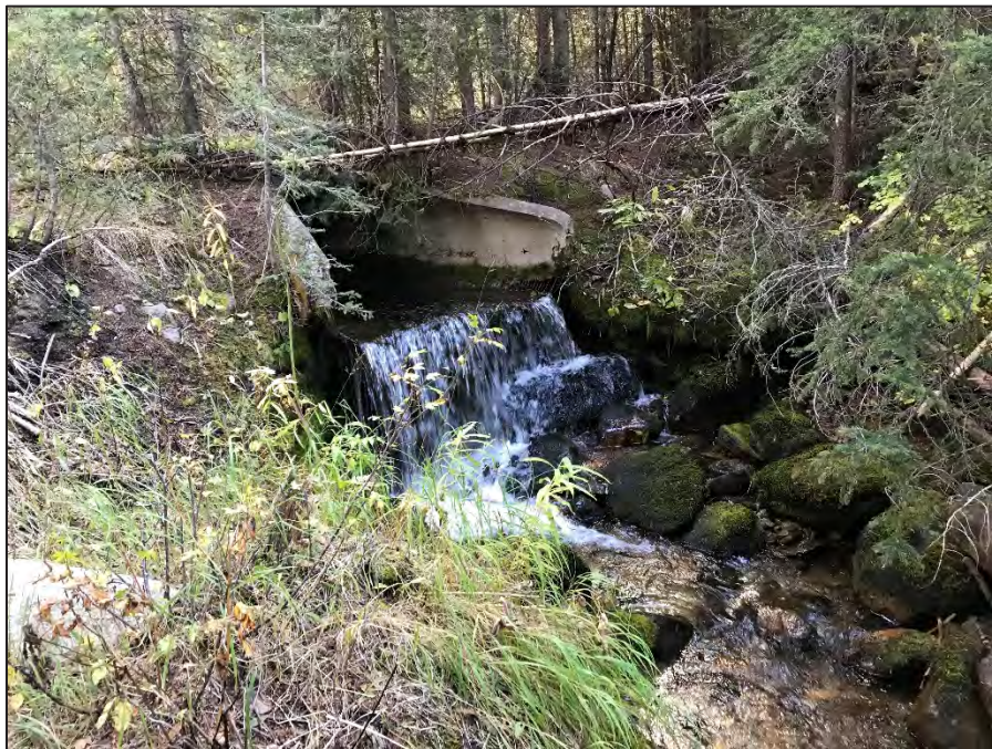
Figure 2 – Existing RCP outlet
