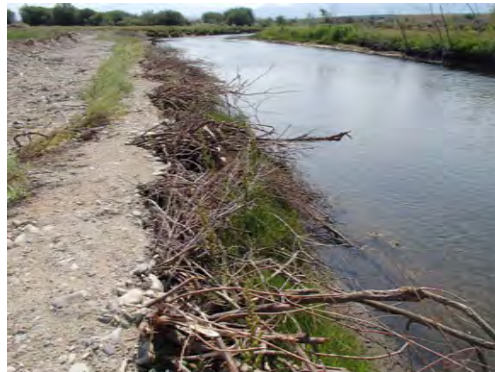
EXAMPLES OF WOODY DEBRIS MATRIX STREAMBANK TREATMENTS
