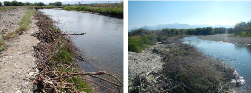
EXAMPLES OF WOODY DEBRIS MATRIX STREAMBANK TREATMENTS
