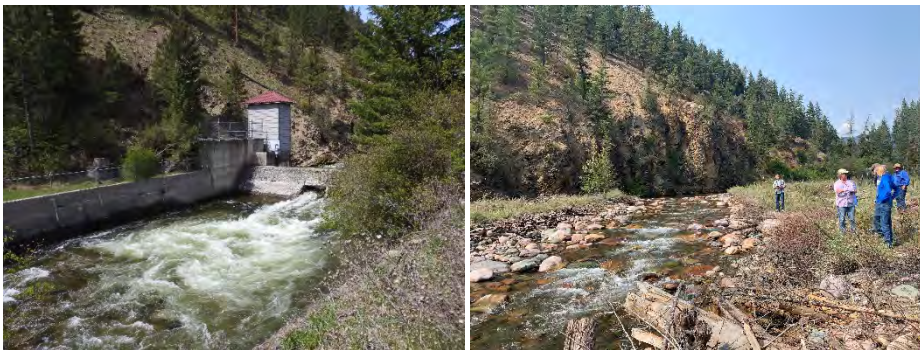
FIGURE 35. RATTLESNAKE DAM PRIOR TO REMOVAL (L) AND IN 2021 (R).
