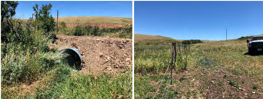
FIGURE 8. BIG OTTER CREEK AFTER CONSTRUCTION, CULVERT (L) AND FENCE (R) INSTALLED.
