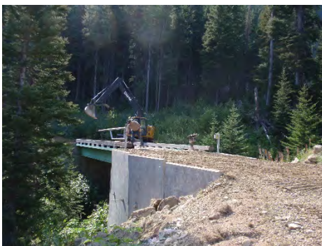
FIGURE 43. SOUTH WOODWARD BRIDGE REPAIR, DURING CONSTRUCTION (2013).
