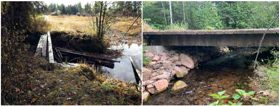
FIGURE 40. SHANLEY CREEK CROSSING BEFORE CONSTRUCTION (L) AND IN 2021 (R).
