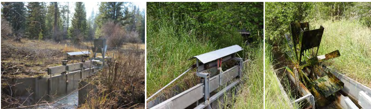
FIGURE 39. SHANLEY CREEK FISH SCREEN AFTER CONSTRUCTION (2016, L) AND IN 2021 (MIDDLE, R).
