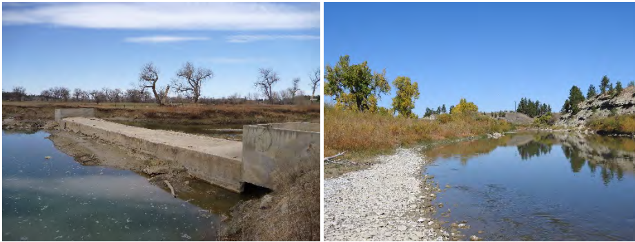
FIGURE 29. THE EGGE DIVERSION BEFORE REMOVAL (L) AND IN 2021 (R).
