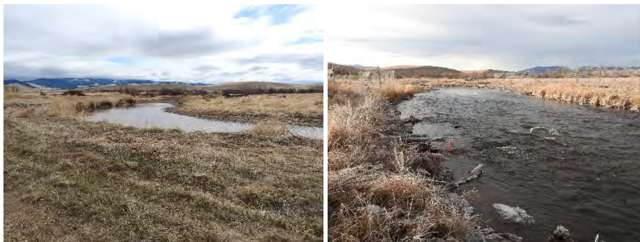
FIGURE 12. FLINT CREEK STREAM RESTORATION BEFORE (L) AND AFTER (R) CONSTRUCTION.
