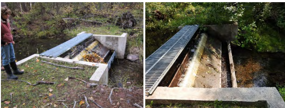
FIGURE 24. DICK CREEK FISH SCREEN IN 2011 (L) AND IN 2021 (R).
