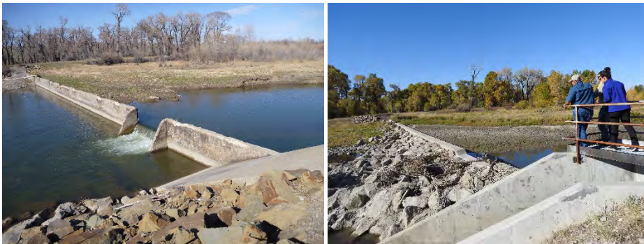
FIGURE 23. DEADMAN'S BASIN DIVERSION DAM BEFORE CONSTRUCTION (L) AND IN 2021 (R).
