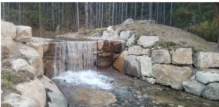
FIGURE 4. ANDRUS CREEK FISH BARRIER, AFTER COMPLETION.
