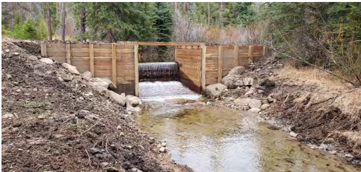
FIGURE 10. DOOLITTLE CREEK FISH BARRIER AFTER CONSTRUCTION.
