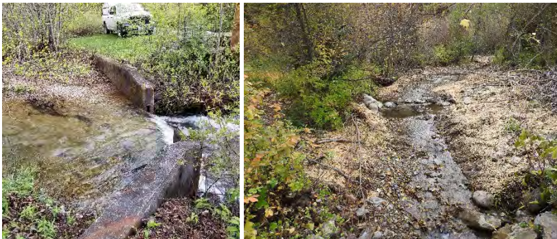
FIGURE 13. HALL CREEK FISH BARRIER BEFORE (L) AND AFTER (R) REMOVAL.
