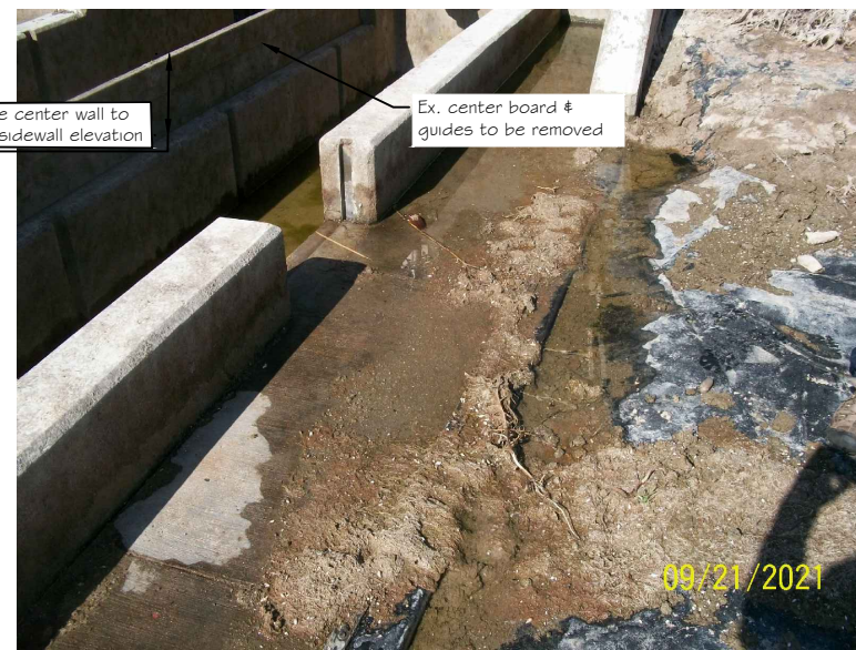
Ex. Kettle Center Wall (to be raised)
