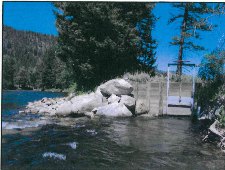
Diversion (left) for ditch at RM 50.5 on Rock Creek and headgate (right), surveyed in 2010 and 2011.
