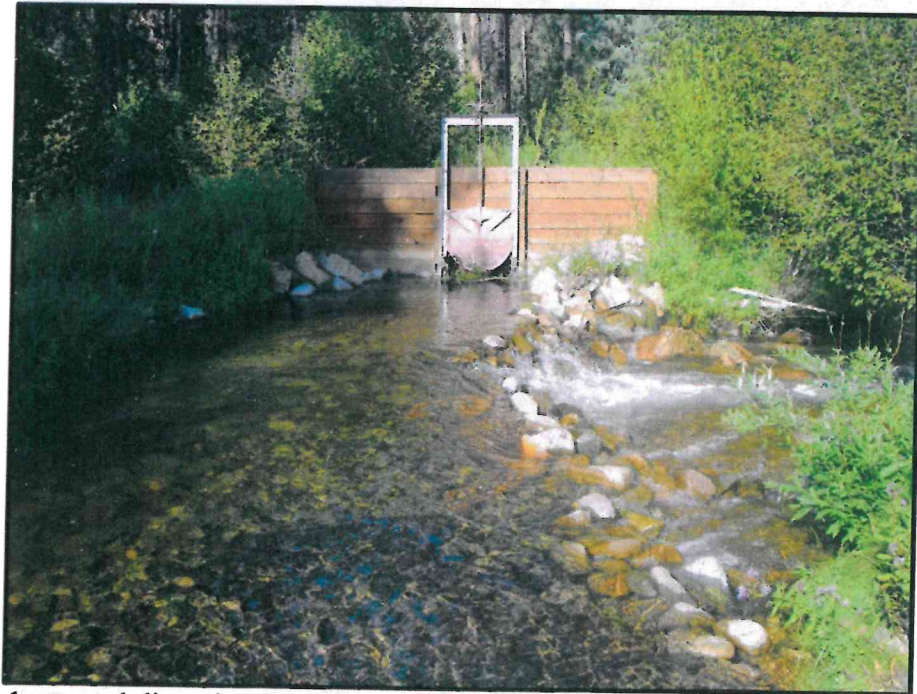
Headgate and diversion for ditch at RM 0.3 on Stony Creek, surveyed in 2009.
