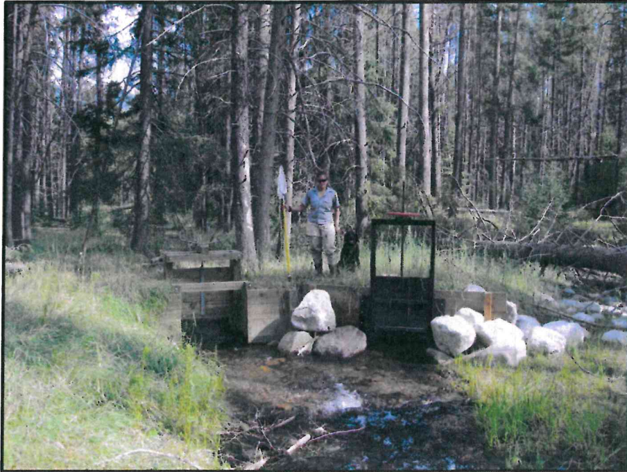
Check dam and headgate for ditch at RM 0.9 on Beaver Creek, surveyed in 2009.
