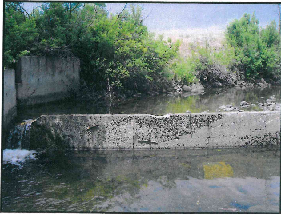
Concrete diversion for ditch at RM 5.5 on Cottonwood Creek, surveyed 2009. This structure was replaced with a rock v-weir structure in fall 2011.
