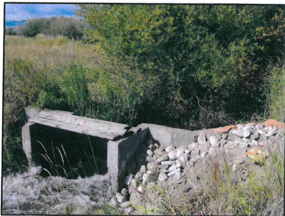
Check-dam (left) and headgate (right) for ditch at RM 4.7 on Dempsey Creek, surveyed in 2010.
