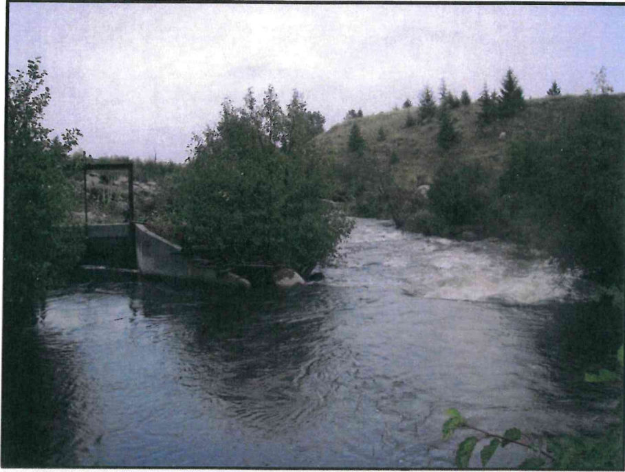
Headgate (left) and diversion (right) for ditch at RM 7.5 on Racetrack Creek, surveyed in 2010.
