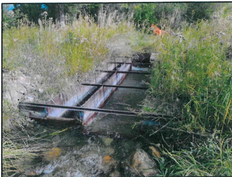
View of the fish screen in place on ditch at RM 1.1, surveyed in 2010.
