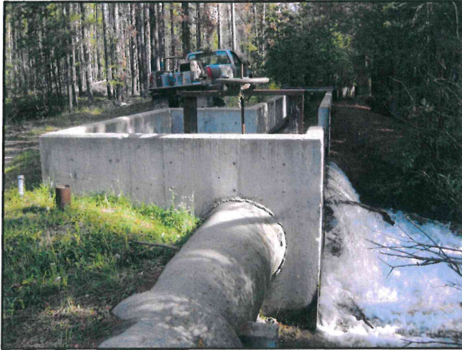
View of the water control structure on Storm Lake Creek. Pipe in the foreground leads to Warm Springs Creek and spill on the right leads to Silver Lake.
