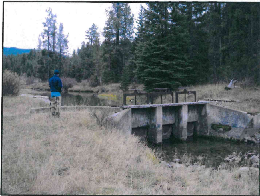
Headgate for Flint Creek Main Canal.
