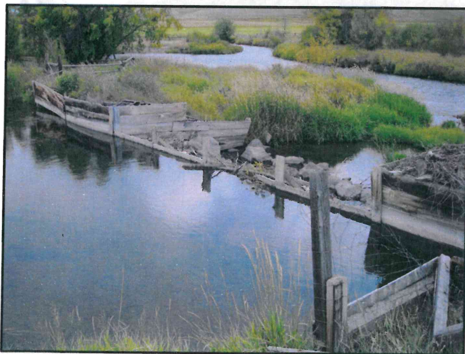
Cottonwood Creek diversion and secondary headgate (right) on Kohrs-Manning ditch (approximately 0.25 mi below headgate).
