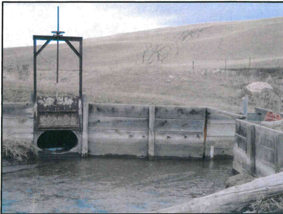
Headgate and check-dam (right) for ditch at RM 1.1 ditch on Gird Creek.
