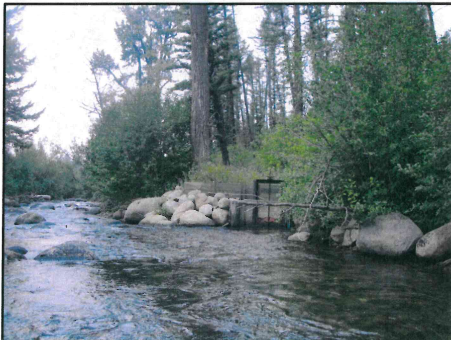
Headgate for ditch at RM 0.9 ditch on Boulder Creek, surveyed in 2009 and 2010.
