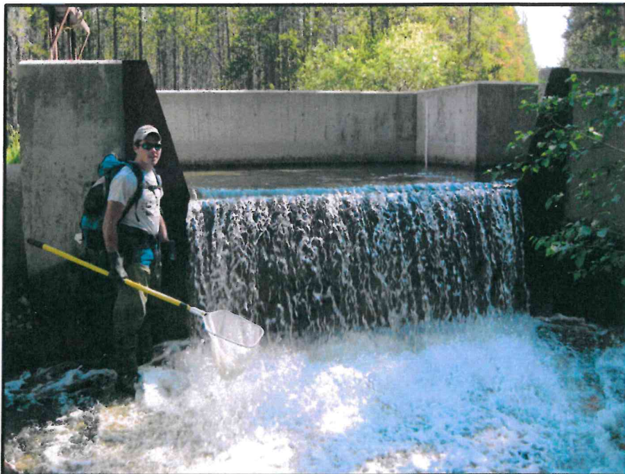
View of the vertical barrier on the Storm Lake Creek structure.
