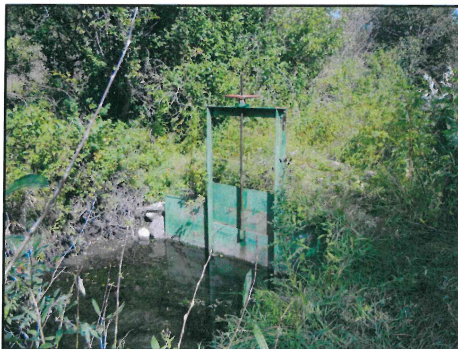
Headgate for ditch at RM 3.6 on Gold Creek, surveyed in 2010.
