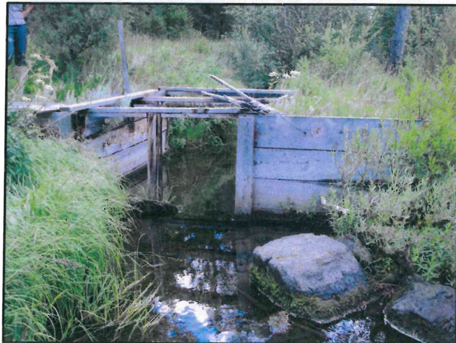
Headgate for ditch at RM 4.2 on West Fork Rock Creek, surveyed in 2010.
