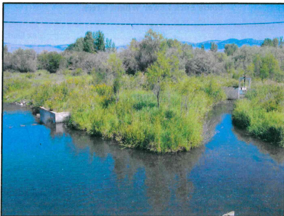
Diversion (left) and headgate (right) of the diversion near Hall, MT.
