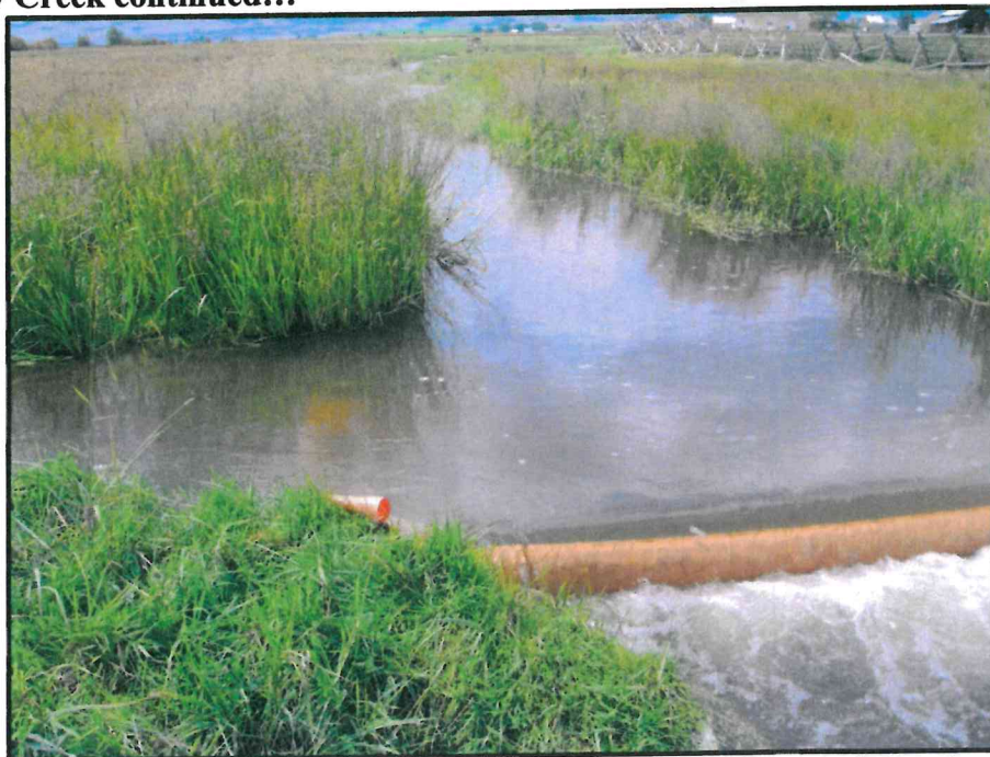
Temporary diversion for ditch (left) at RM 2.0 on Dempsey Creek.
