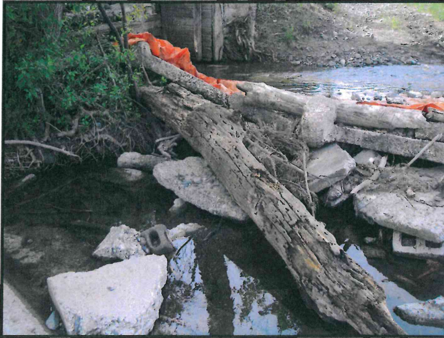
Diversion for ditch at RM 3.5 on Cottonwood Creek, surveyed 2009.
