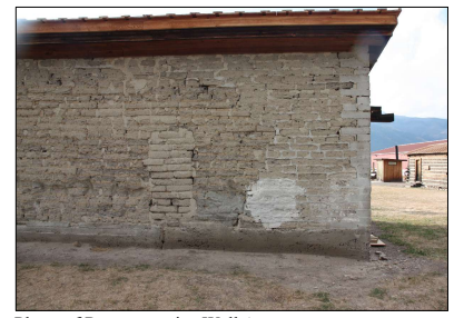
Photo of Representative Wall Area North End of East Wall
