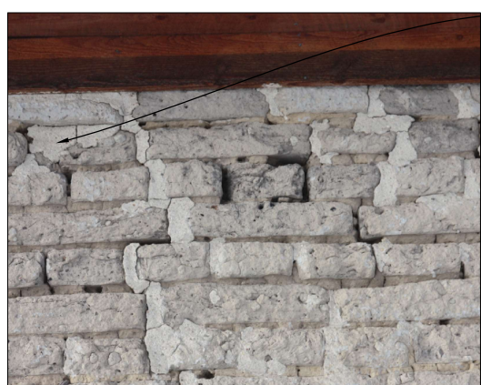
5 CONCRETE PATCH REMOVAL
