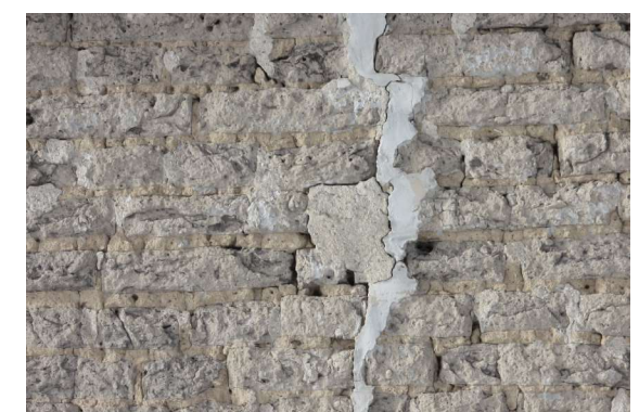
6 CONCRETE FILL Not to Scale THIS PHOTO SHOWS PAINTED CONCRETE FILL SCHEDULED FOR REMOVAL PER NOTE R10 ON SHEET 5.
