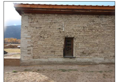
Photo of Representative Wall Area South End of East Wall
