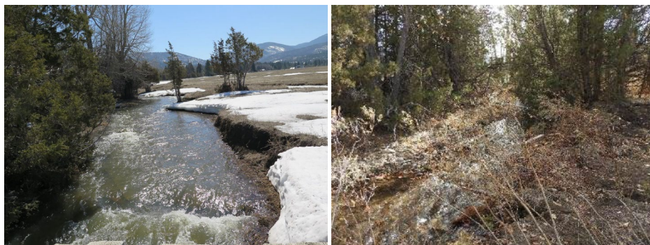
FIGURE 24. POORMAN CREEK BEFORE (L) AND AFTER (R) CONSTRUCTION. PHOTOS COURTESY OF BIG BLACKFOOT CHAPTER OF TROUT UNLIMITED AND FWP.
