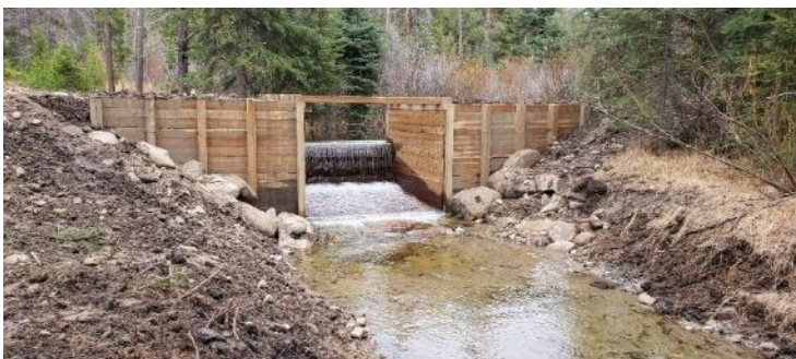
FIGURE 15. DOOLITTLE CREEK FISH BARRIER AFTER CONSTRUCTION.
