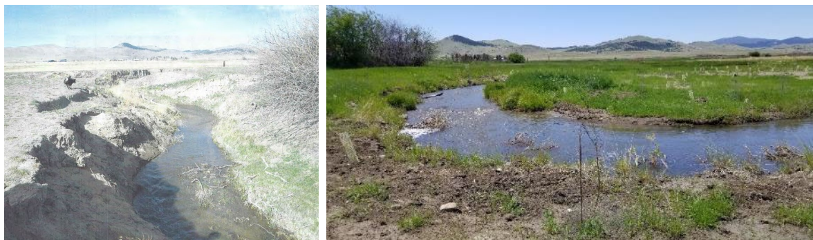
FIGURE 25. SEVENMILE CREEK BEFORE (L) AND AFTER (R) CONSTRUCTION. PHOTOS COURTESY OF PRICKLY PEAR LAND TRUST.
