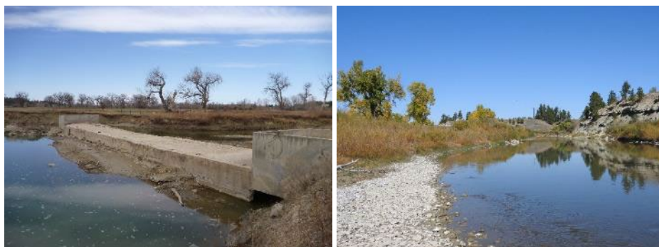
FIGURE 35. THE EGGE DIVERSION BEFORE REMOVAL (L) AND IN 2021 (R).
