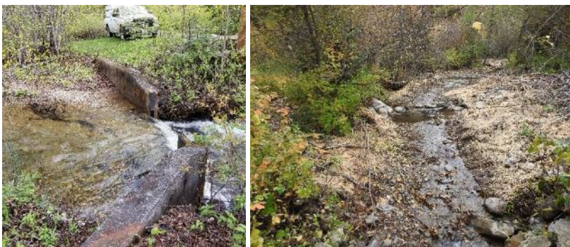
FIGURE 18. HALL CREEK FISH BARRIER BEFORE (L) AND AFTER (R) REMOVAL.
