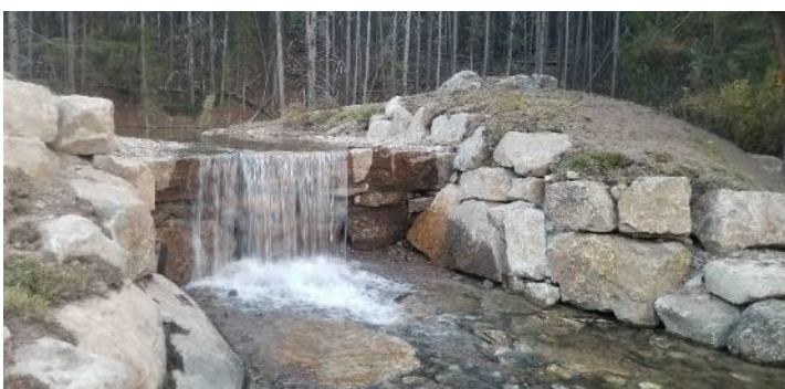
FIGURE 8. ANDRUS CREEK FISH BARRIER, AFTER COMPLETION.
