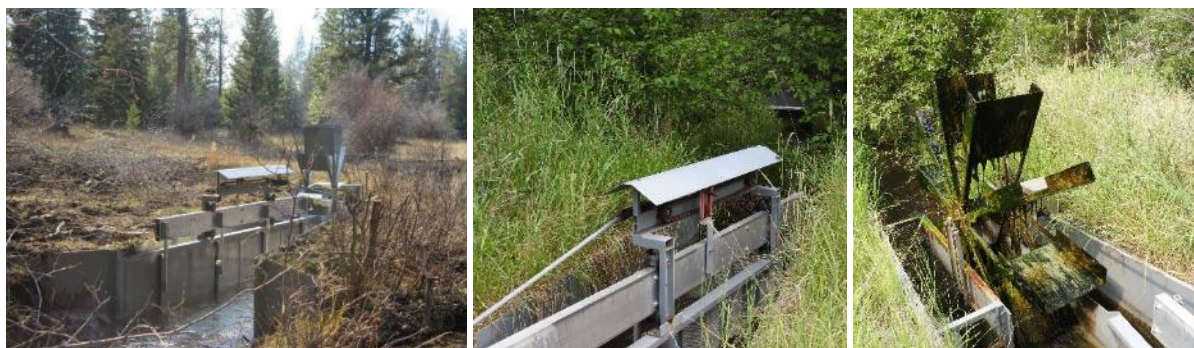
FIGURE 46. SHANLEY CREEK FISH SCREEN AFTER CONSTRUCTION (2016, L) AND IN 2021 (MIDDLE, R).
