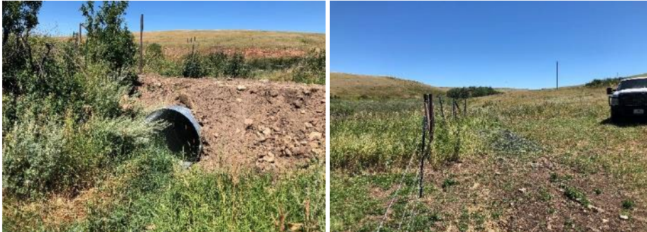
FIGURE 13. BIG OTTER CREEK AFTER CONSTRUCTION, CULVERT (L) AND FENCE (R) INSTALLED.
