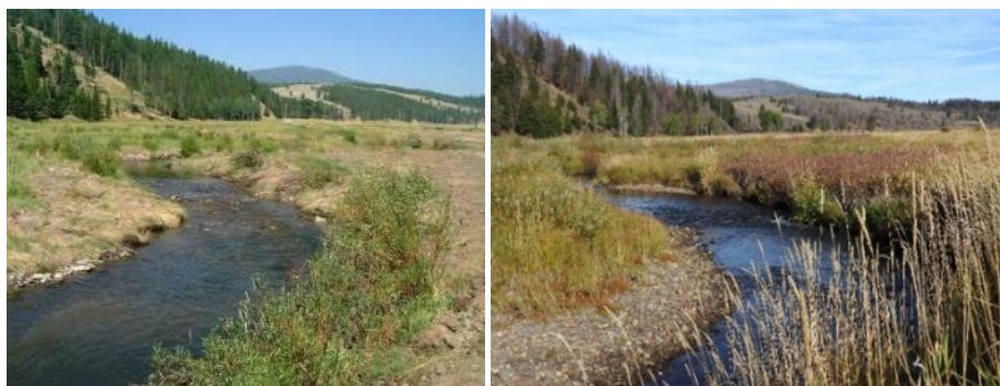
FIGURE 53. UPPER WILLOW CREEK AFTER CONSTRUCTION (2005, L) AND IN 2021 (R).
