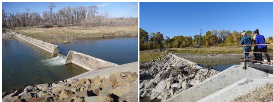
FIGURE 29. DEADMAN'S BASIN DIVERSION DAM BEFORE CONSTRUCTION (L) AND IN 2021 (R).
