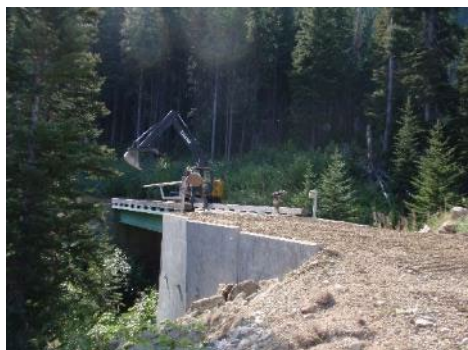
FIGURE 50. SOUTH WOODWARD BRIDGE REPAIR, DURING CONSTRUCTION (2013).
