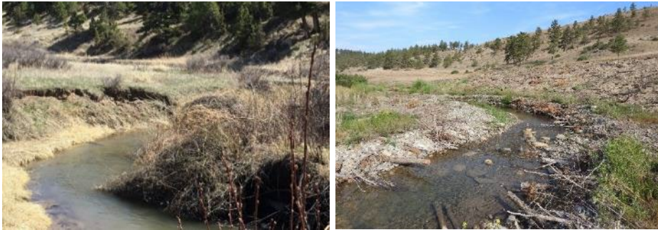
FIGURE 12. BEAVER CREEK CHANNEL RECONSTRUCTION BEFORE (L) AND AFTER (R) CONSTRUCTION. PHOTOS COURTESY OF THE US FOREST SERVICE AND FWP.
