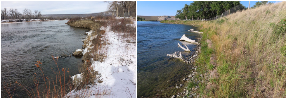
FIGURE 34. MARIAS RIVER BEFORE CONSTRUCTION (L) AND IN 2021 (R).
