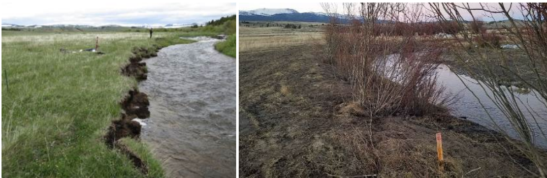
FIGURE 20. LOWER FRENCH CREEK RESTORATION BEFORE (L) AND AFTER (R) CONSTRUCTION.
