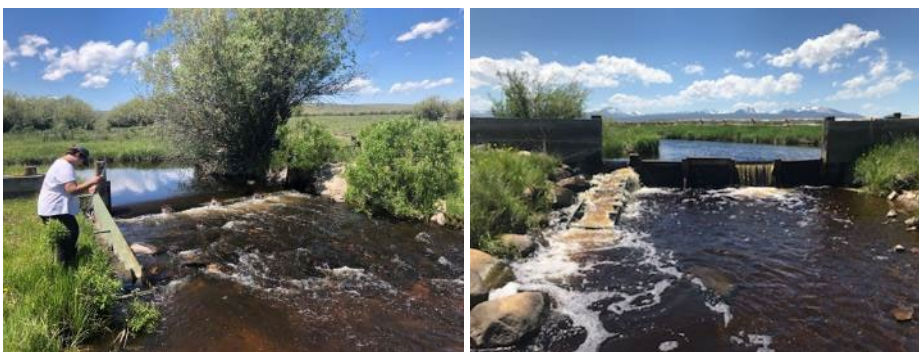
FIGURE 45. PHOTOS OF SEVERAL OF THE IRRIGATION DIVERSIONS WITH DENIL FISH LADDERS.
