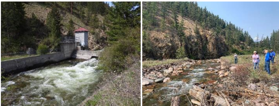
FIGURE 41. RATTLESNAKE DAM PRIOR TO REMOVAL (L) AND IN 2021 (R).
