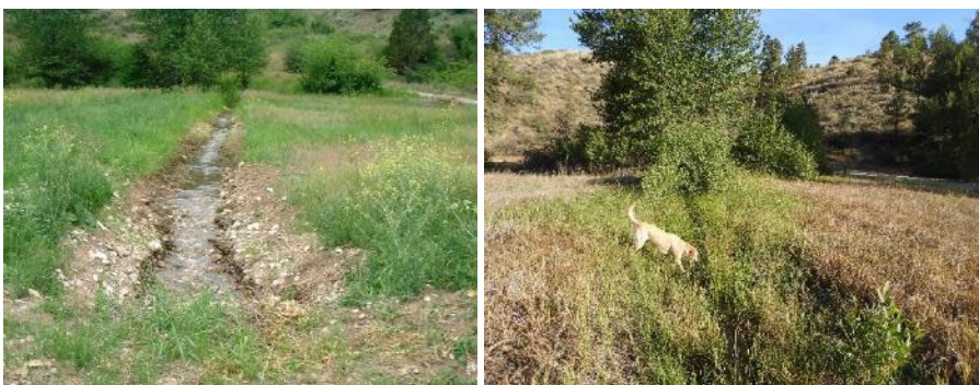
FIGURE 26. THE BEAVER CREEK DIVERSION PROJECT AFTER COMPLETION (2003, L) AND IN 2021 (R).
