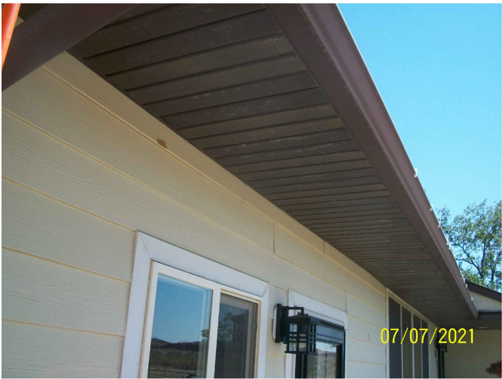
House #101 eaves, soffit & window trim
