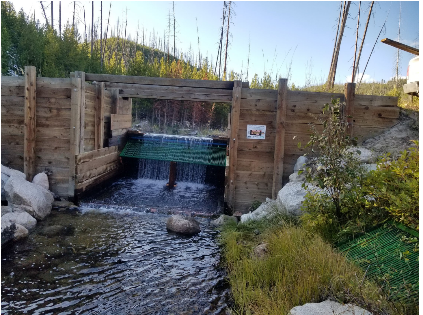
Figure 2. Bender Creek fish barrier constructed in 2017 which would be similar to the barrier proposed on Bryant Creek.
