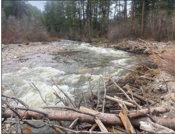
Example treatment using logs and woody debris
