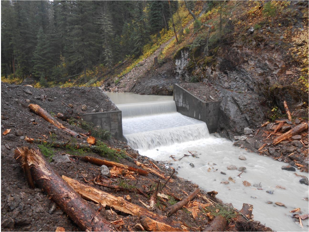
Photo 3. Upstream view of the Cabin Creek fish barrier. The cast-in-place structure utilizes a double drop design to prevent backwatering of the splashpad and wing walls to confine flood flows to the barrier. This ensures that the barrier prevents upstream fish passage during floods. Stream width and valley width and bedrock confinement are similar to the proposed Mill Creek fish barrier site.
