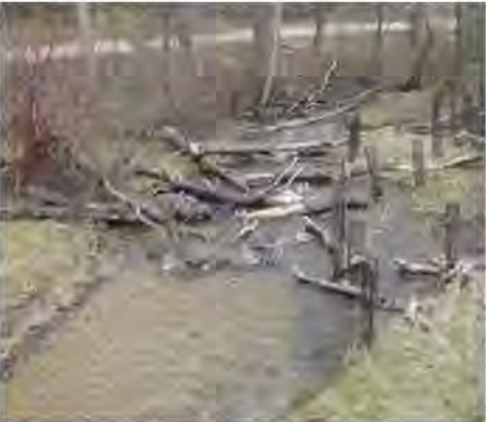
Constructed Large Wood Habitat Structures
