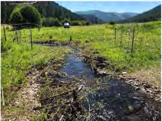
Constructed Woody Debris Matrix streambank treatments
