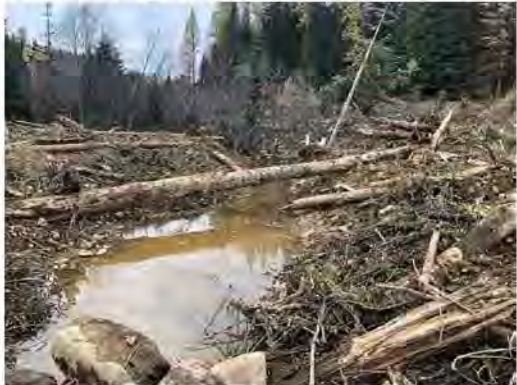
Floodplain wetland enhancement with surface roughness and woody debris
