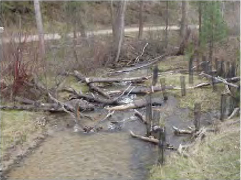
Examples of Large Wood Habitat Structures
