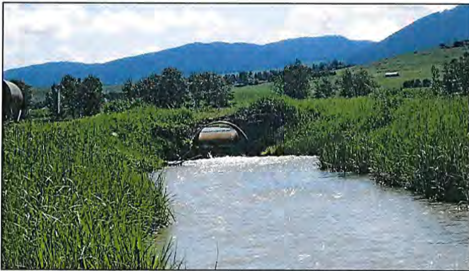
Figure 1. Diversion and partial fish barrier on Wilson Creek
