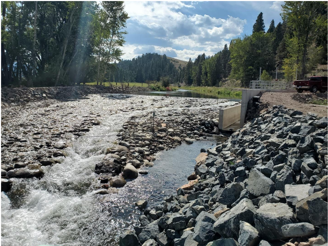
Photo 1. The fishway and constructed riffle at the Private Users diversion. The PIT antennas are housed in PVC pipe and can be seen near the bottom and top of the fishway.
