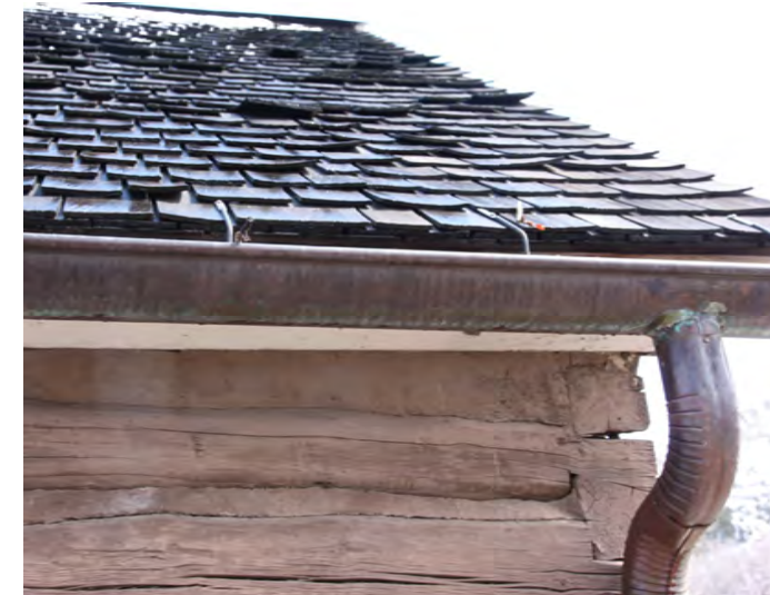
5 Manager's House - Gutter Photograph - Not to Scale
