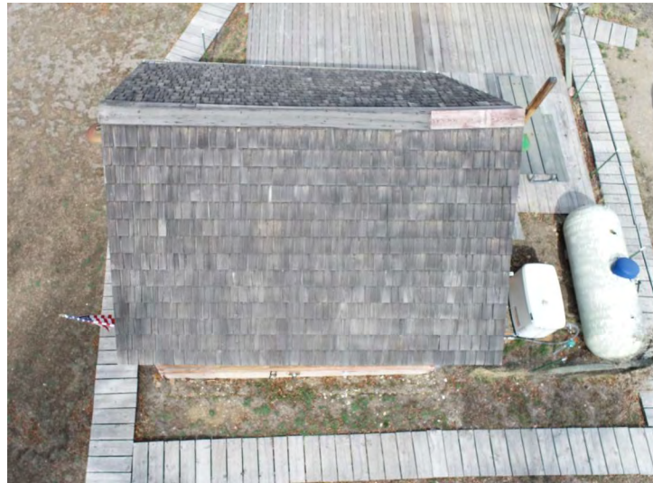
3 Manager's Office - Roof Aerial Photograph From the North - Not to Scale
