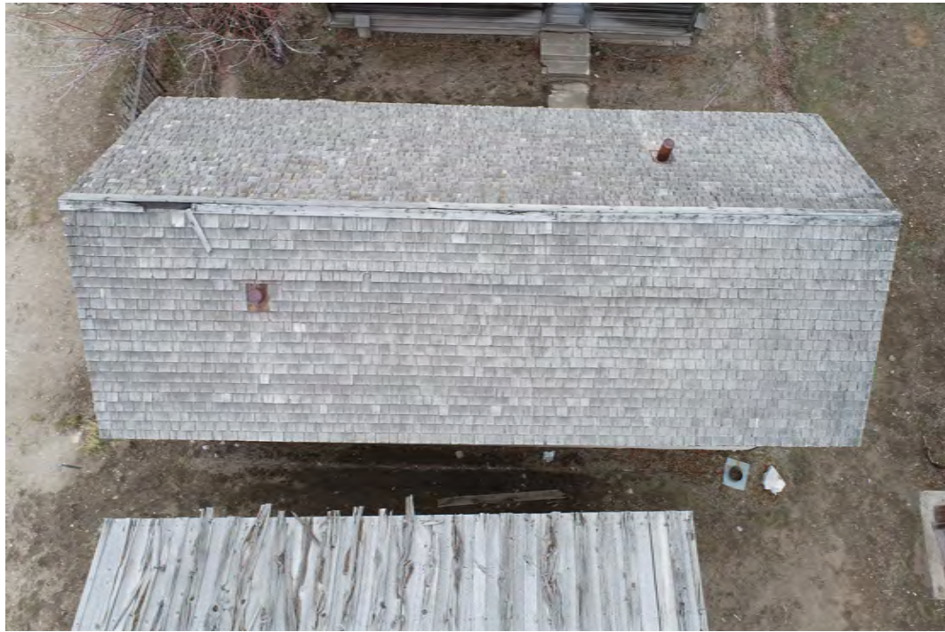
3 Firehouse - Roof Photo from the West Aerial Photograph - Not to Scale
