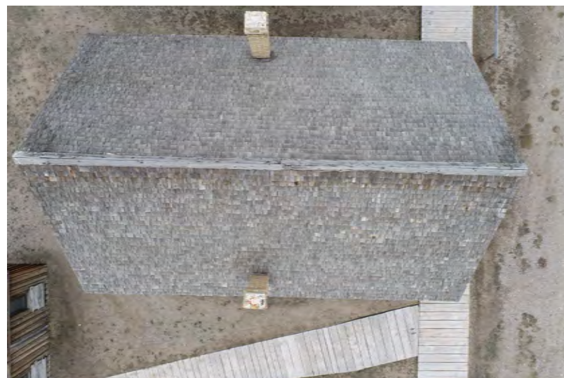
1 Gibson House - Roof Photo from East
