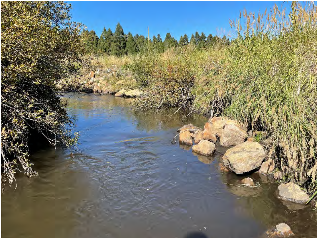
Second section of aging rock rip-rap, along incised section, looking West, Station 14+50, 9-20-22.
