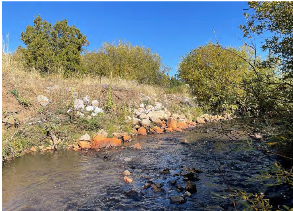
Aging rock rip-rap, along incised section, downstream of rock riffle, looking North, Station 12+00, 9-20-22.
