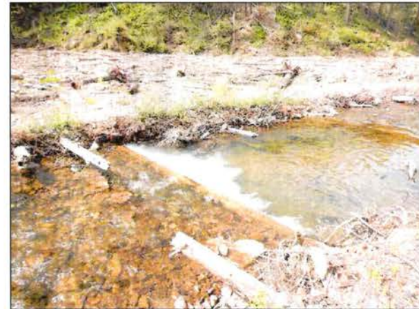
EXAMPLE OF A CONSTRUCTED LOG STEP POOL
