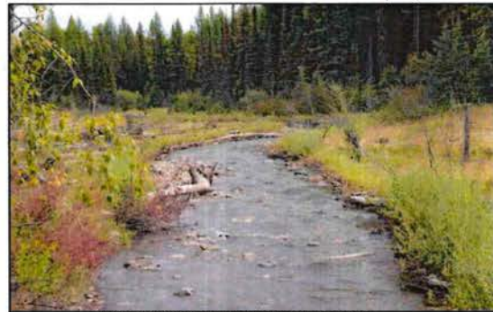
TYPICAL CONSTRUCTED STREAMBED THROUGH A RIFFLE FEATURE
