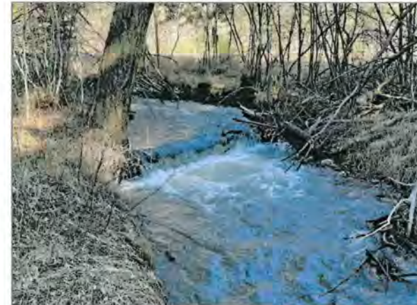
EXAMPLE OF A CONSTRUCTED LOG STEP POOL
