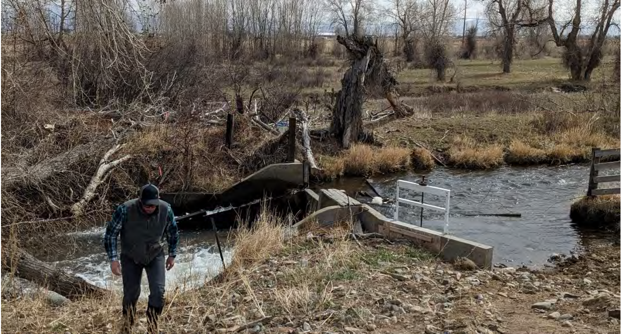
Photo 1. Diversion structure and fixed-wheel headgate (June 9, 2022; 110 CFS).
