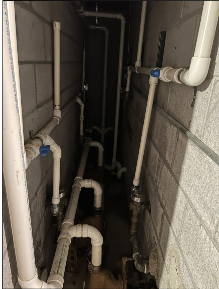
Comfort Station Access Room
