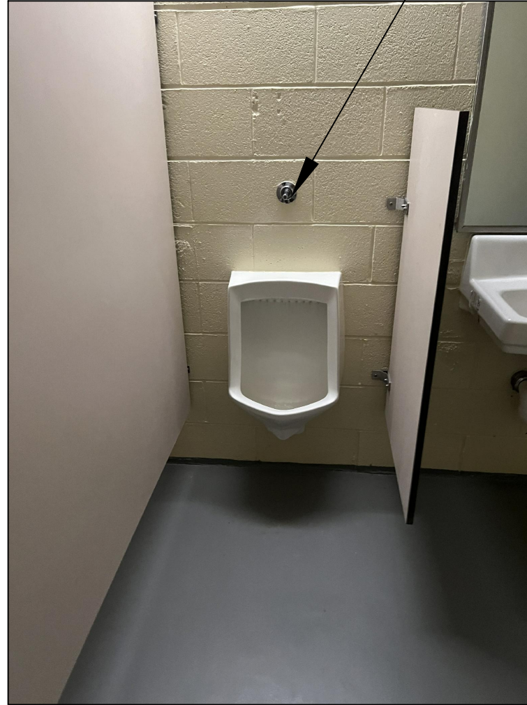
Urinal Fixture Replacement
