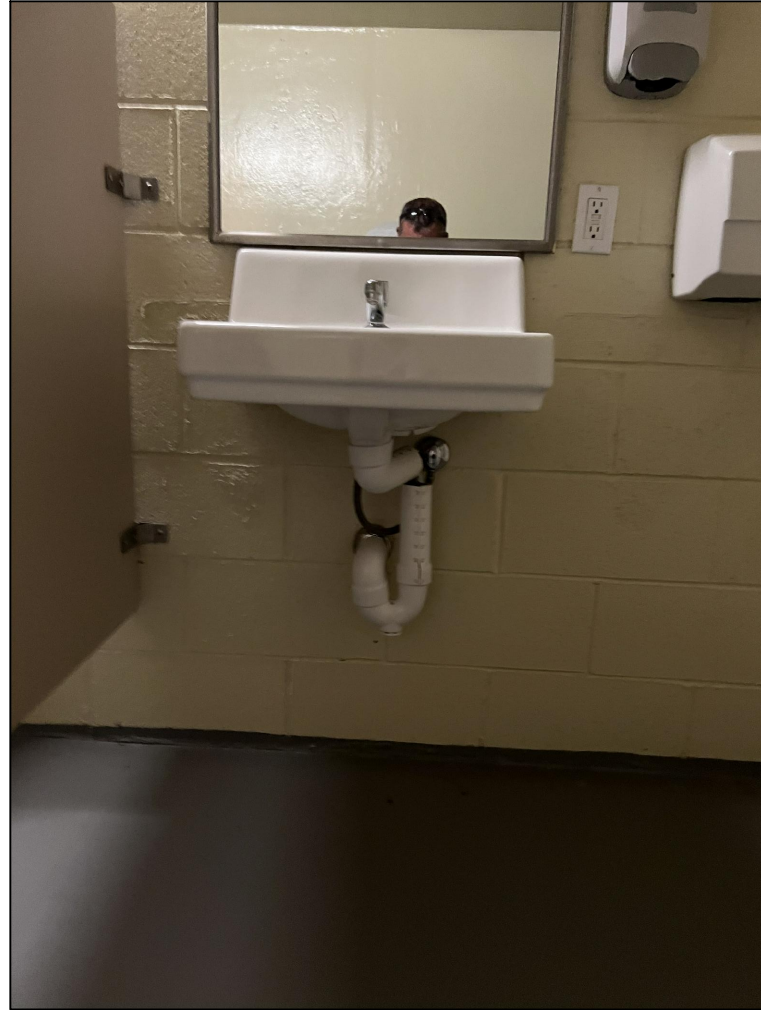
Sink Fixture Replacement
