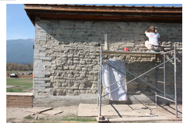
Photo of Representative Wall Area South End of East Wall
