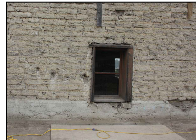
Photo of Representative Wall Area Window into Room #102, at East Wall
