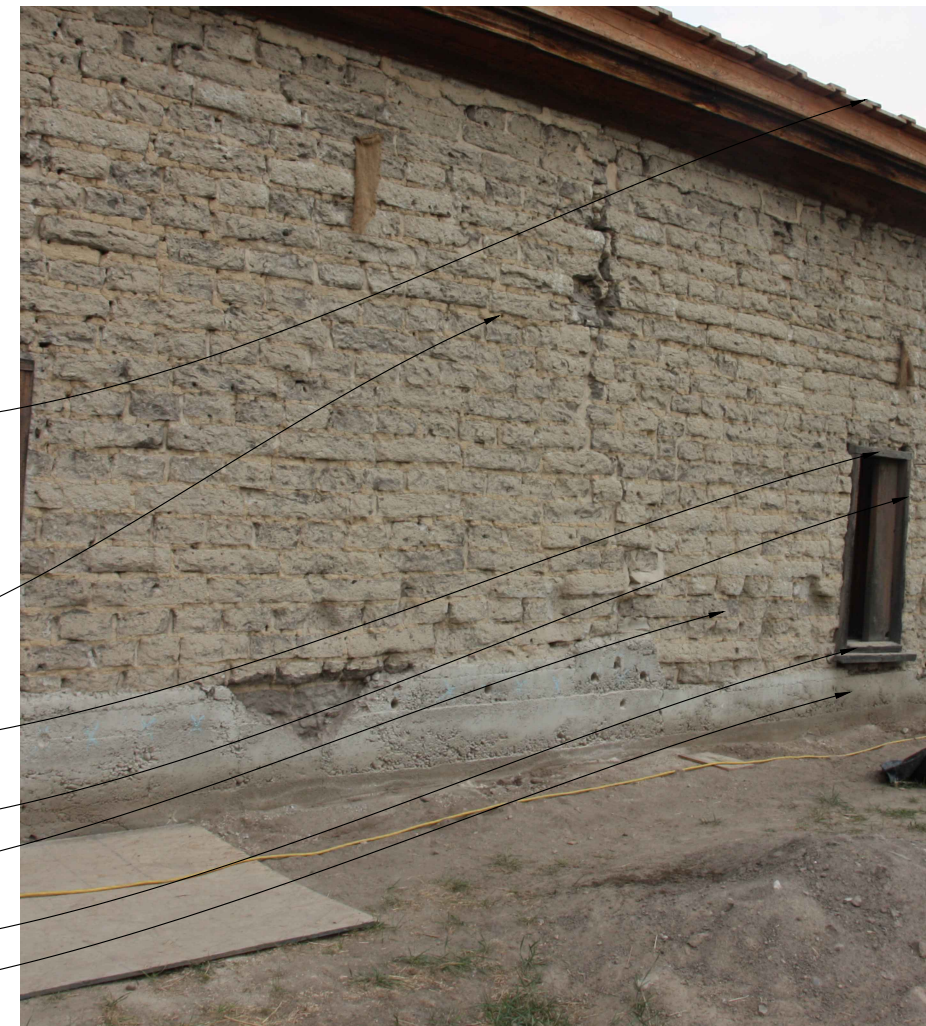
3 EAST ELEVATION PHOTOGRAPH Not to Scale
