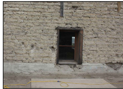
Photo of Representative Wall Area Window into Room #102, at East Wall
