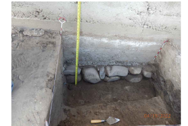
Photo of Representative Test Pit at East Wall Showing stone foundation and concrete plinth above
