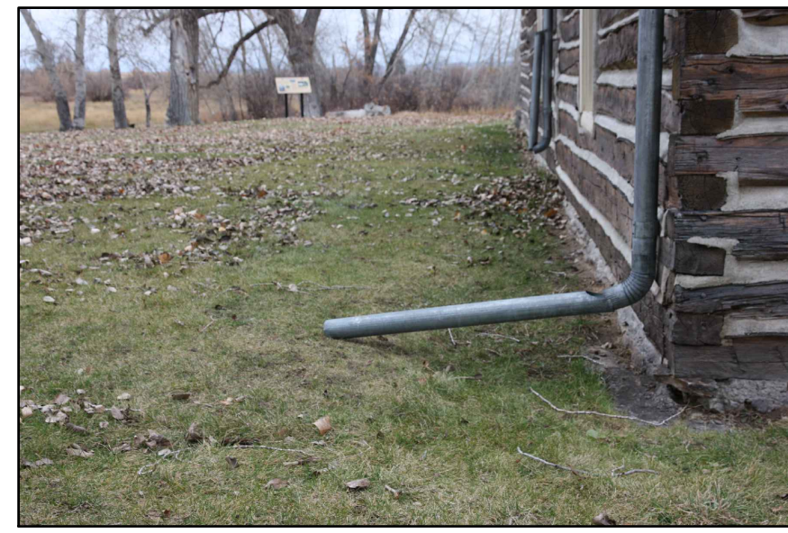
3 A3 CHIEF'S HOUSE, EARTH SLOPING DOWN TOWARDS NORTH SIDE OF BUILDING
