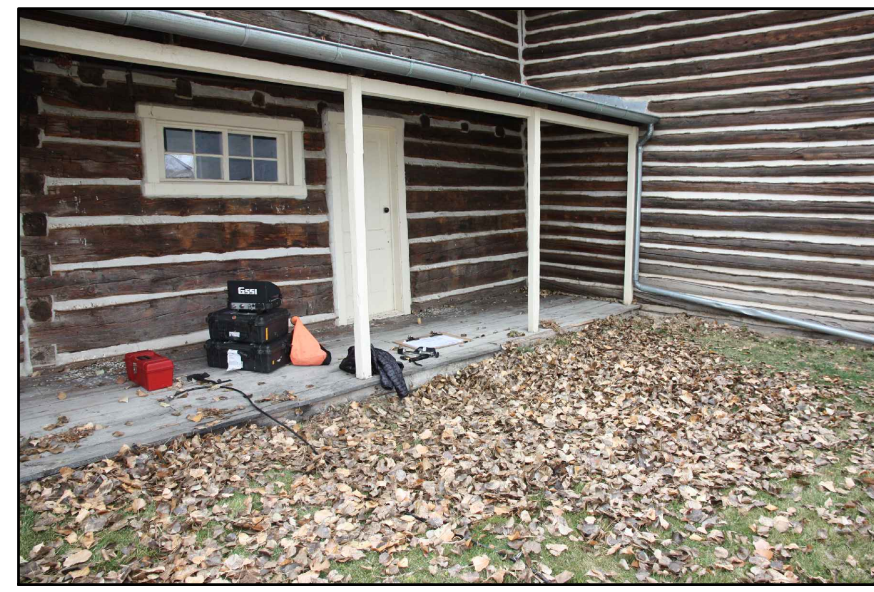
2 A3 CHIEF'S HOUSE LEAVES PILED UP IN FRONT OF SOUTH PORCH
