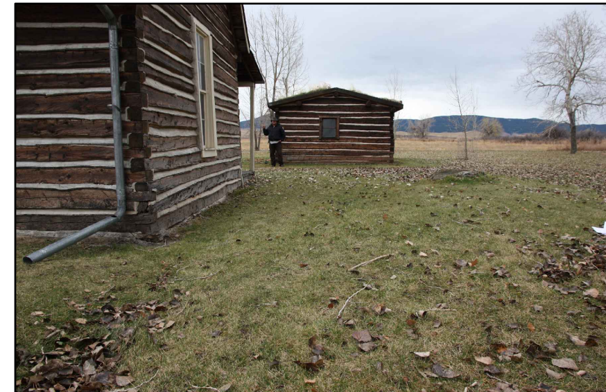
8 A3 NORTHWEST CORNER, SHOWING EARTH SLOPING DOWN TOWARDS WEST SIDE ON BUILDINGS
