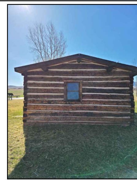
STORE EXTERIOR, NORTH ELEVATION
