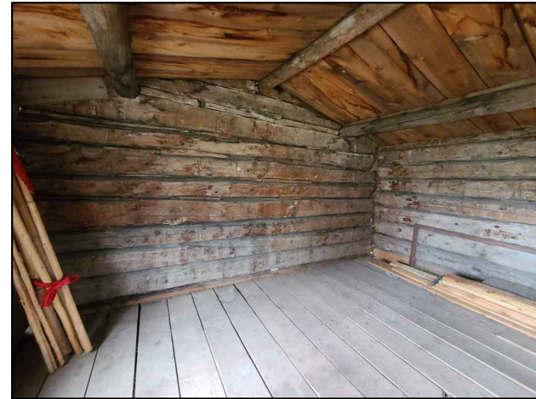
STORE INTERIOR, LOOKING SOUTHWEST
