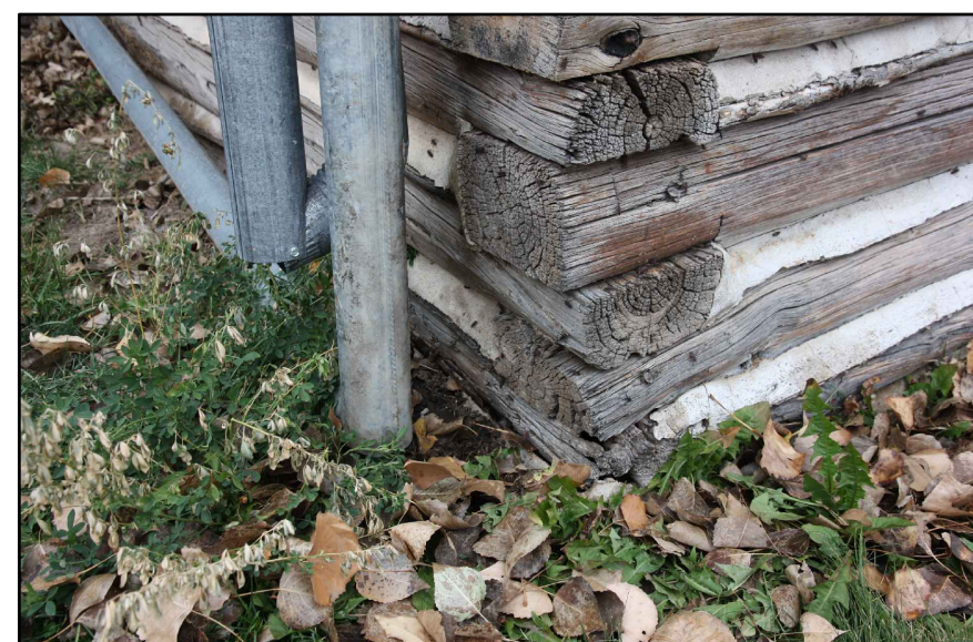
CHIEF'S HOUSE DOWNSPOUT AT SOUTHWEST CORNER
