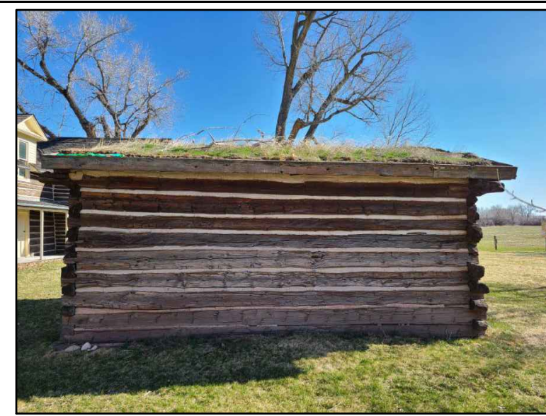
STORE EXTERIOR, WEST ELEVATION
