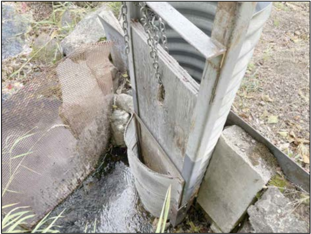
SITE PHOTO: VIEW OF EXISTING HEADGATE, SCREEN MATERIAL AND STEEL HEADWALL
