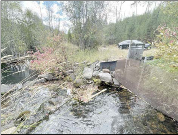
SITE PHOTO: VIEW OF EXISTING DIVERSION AND SCREENED HEADGATE
