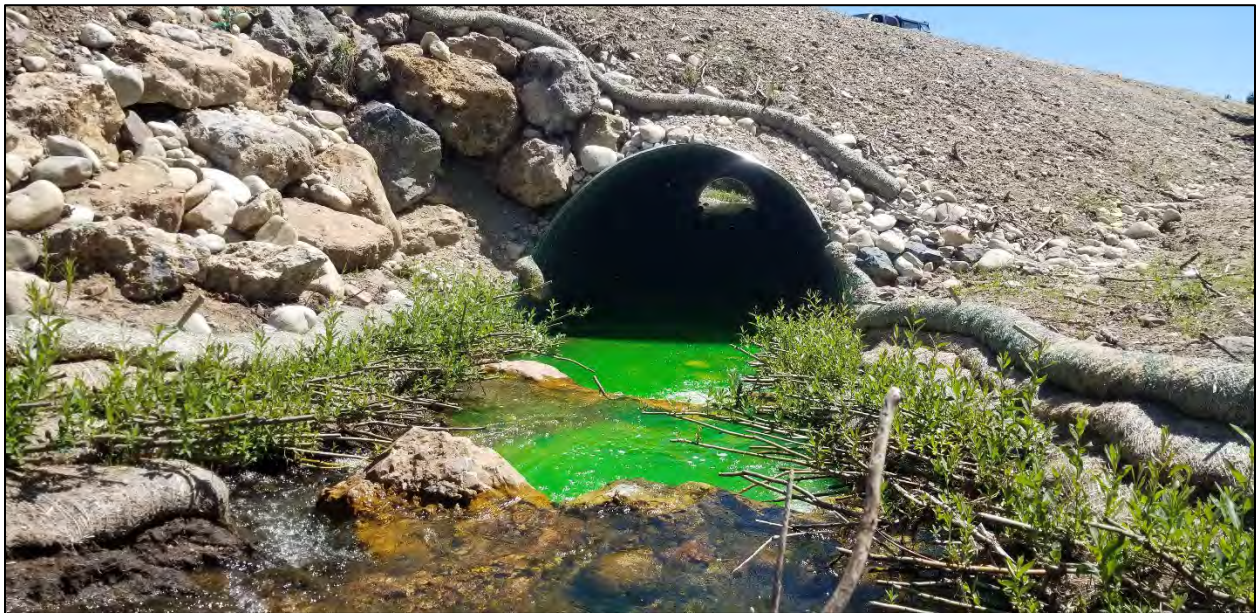
Figure 6. The upstream inlet to the recently completed Oregon Creek culvert replacement (disregard the green rotenone treatments). Note the step-pools leading to the inlet. We will use this step-pool configuration as a reference while installing the Sixmile culvert and to catch appropriate grades.
