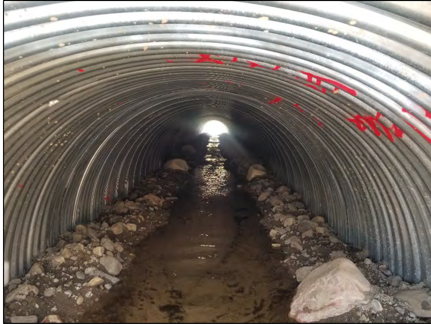
Figure 5. This is a recently completed culvert replacement on Oregon Creek, just downstream of Sixmile Creek. We will use this culvert as an example and reference to the Sixmile Creek replacement. Note the well-mixed alluvium in the culvert bottom and the abundance of fine sediments. This was a considered decision to allow for low summer surface water to flow over the fines instead of through the interstitial spaces of the larger gravels and rocks; to allow for fish passage. We intend to execute the same strategy on the Sixmile replacement.
