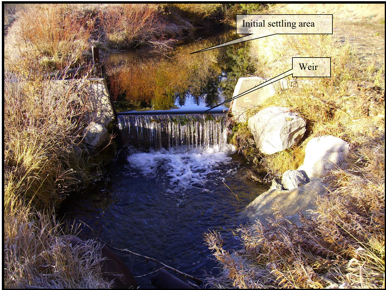
Figure 3. Weir and initial settling area upstream in South Fork North Fork Divide Creek.
