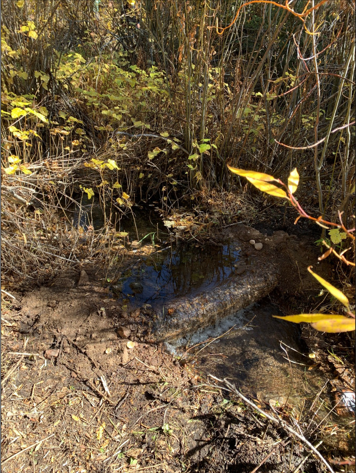
Figure 6. Freshly installed habitat log structure in French Gulch. The same structure design and approach will be used in this proposed First Chance Gulch project.
