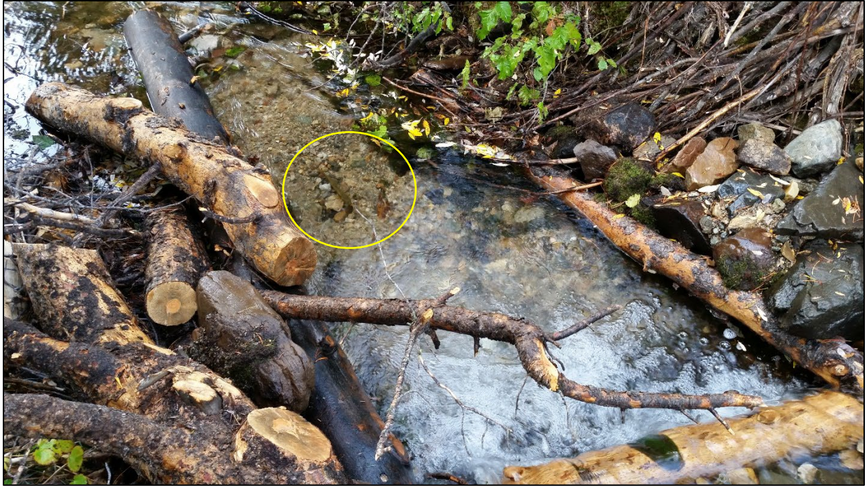
Figure 4. 2016 French Gulch habitat log structure. NOTE the parallel logs used as additional bank side cut habitat. The same technique will be used in strategic locations in First Chance Gulch. Also to NOTE is the fish spawning in the tail-out of the created scour pool (yellow circle) created by the habitat structure.
