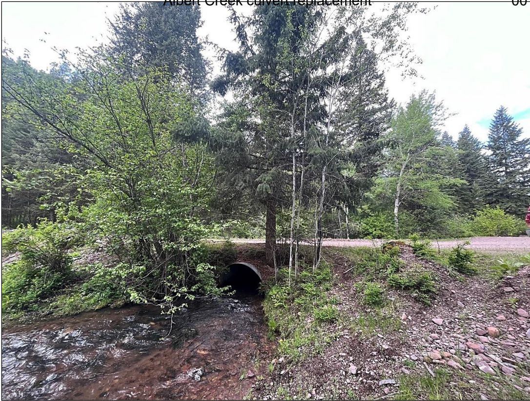
Albert Creek Existing 72"x43" Fish Passage Barrier (Downstream)
