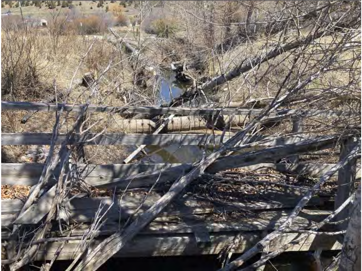
Figure 4- Pre project photo of Fifer Gulch at the beginning of the proposed restoration reach, approximately 1000 feet upstream of Fifer's confluence with Warm Springs Creek. As you can see there are various pieces of old infrastructure that may be inhibiting passage at certain levels.
