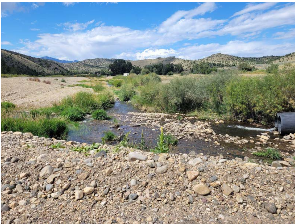
Image 8. Current confluence of Granite Creek and Alder Gulch. The culverts were installed for road stabilization for construction equipment.
