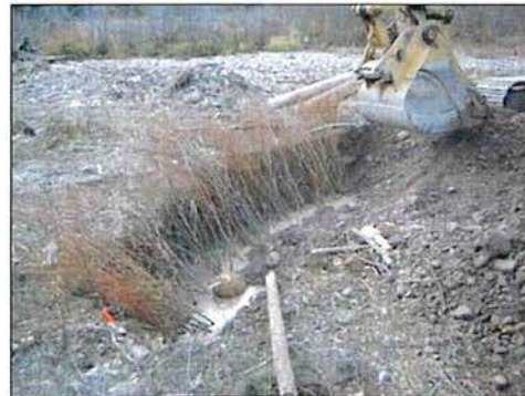
EXAMPLE OF A VEGETATED BRUSH TRENCH INSTALLATION
